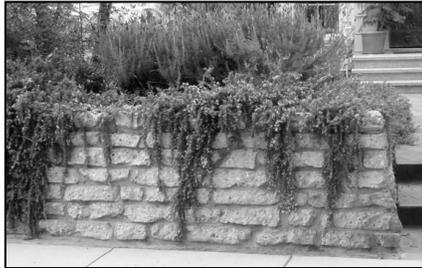
The photo at left shows an example of recycled concrete rip rap (in this case used with mortar to create a garden wall).
