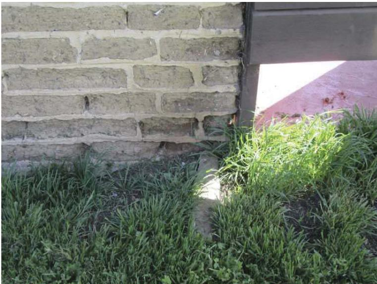
Photo 8. Restroom D showing eroded adobe units at base of wall. Minor regrading to direct the water away from the building will reduce future maintenance.
