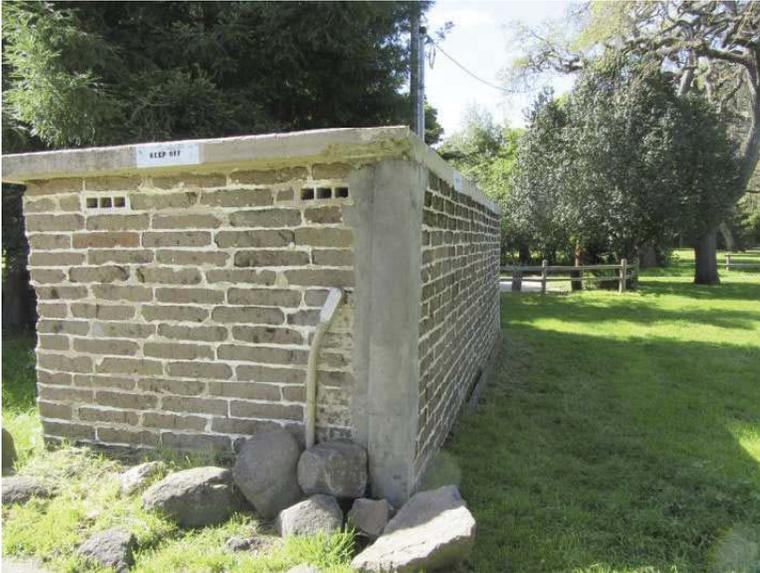
Photo 9. Electrical Equipment building. A low structure now used for the park's electrical equipment. This is the only structure that has a concrete roof.
