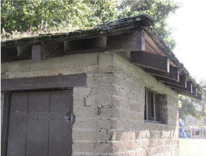
Photo 6. Detail photo of the Maintenance Building showing the concrete bond beam at the top of the wall. There is a crack at the corner that could be previous earthquake damage.
