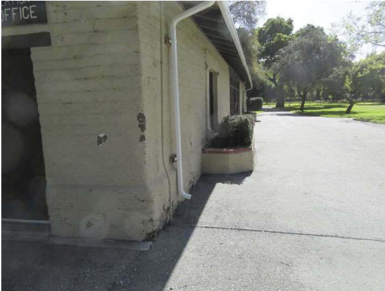
Photo 3. West side of Office Building. The photo shows a planter against the adobe wall. This permits water to enter the adobe blocks and cause erosion.
