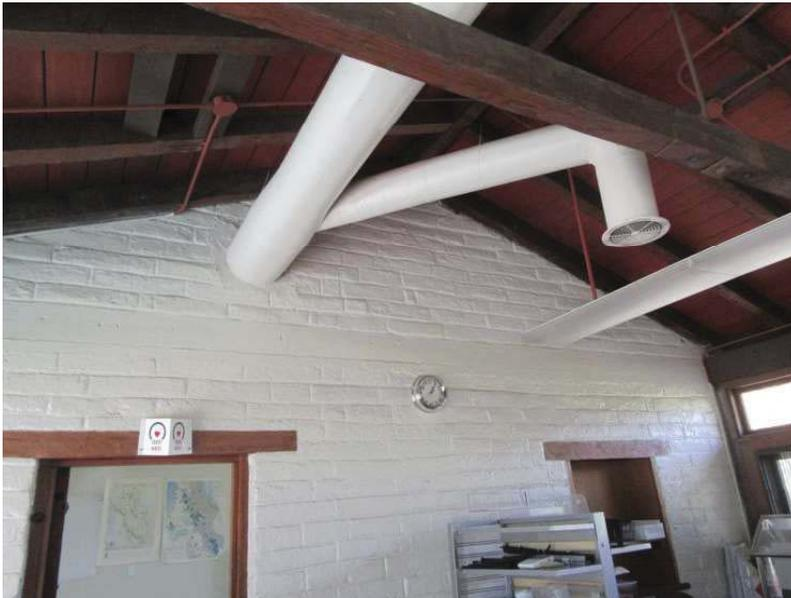
Photo 2. Interior adobe wall showing the gable above the bond beam. Gables act as parapets, which topple in earthquakes. They need to be attached to the roof structure. Roof framing and trusses chords can be seen.
