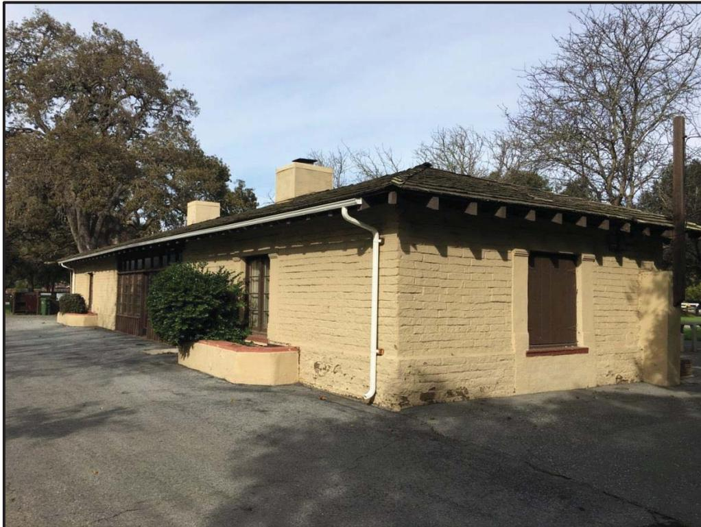
A small rectangular building northeast of the Park Office, the electrical building (MR 8; Figure 11) is constructed of adobe block and has a flat concrete roof. There are punctured concrete blocks below the roofline, likely for ventilation. The building contains a single door which appears to be made of wood with iron hardware. Repairs to the structure are visible at places, such as concrete patching at one of the corners.
