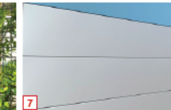
7 EXTERIOR MECHANICAL PENTHOUSE SCREEN METAL SCREEN IN WHITE PAINT FINISH
