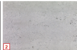
2 EXTERIOR ENVELOPE & WALLS CONCRETE
