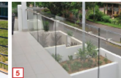
5 EXTERIOR RAILINGS STEEL RAILINGS IN SILVER FINISH AND GLASS BALUSTRADE
