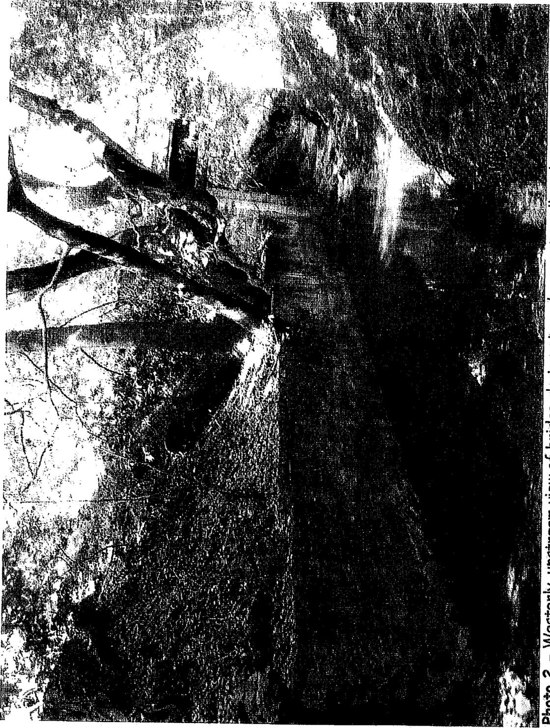
**Photo 2 - Westerly, upstream view of bridge abutments and concrete wall on downstream side. Resistant sandstone lines channel bottom at bridge crossing. Note local bank erosion in distance and end-point erosion at downstream end of wall.**
