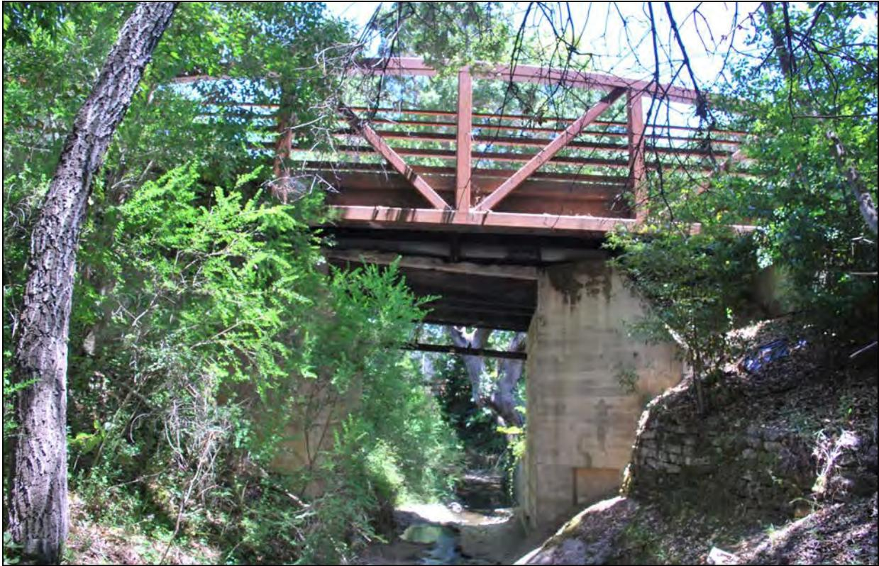
Figure 8: View east towards bridge and south bank – note stacked stone and concrete
