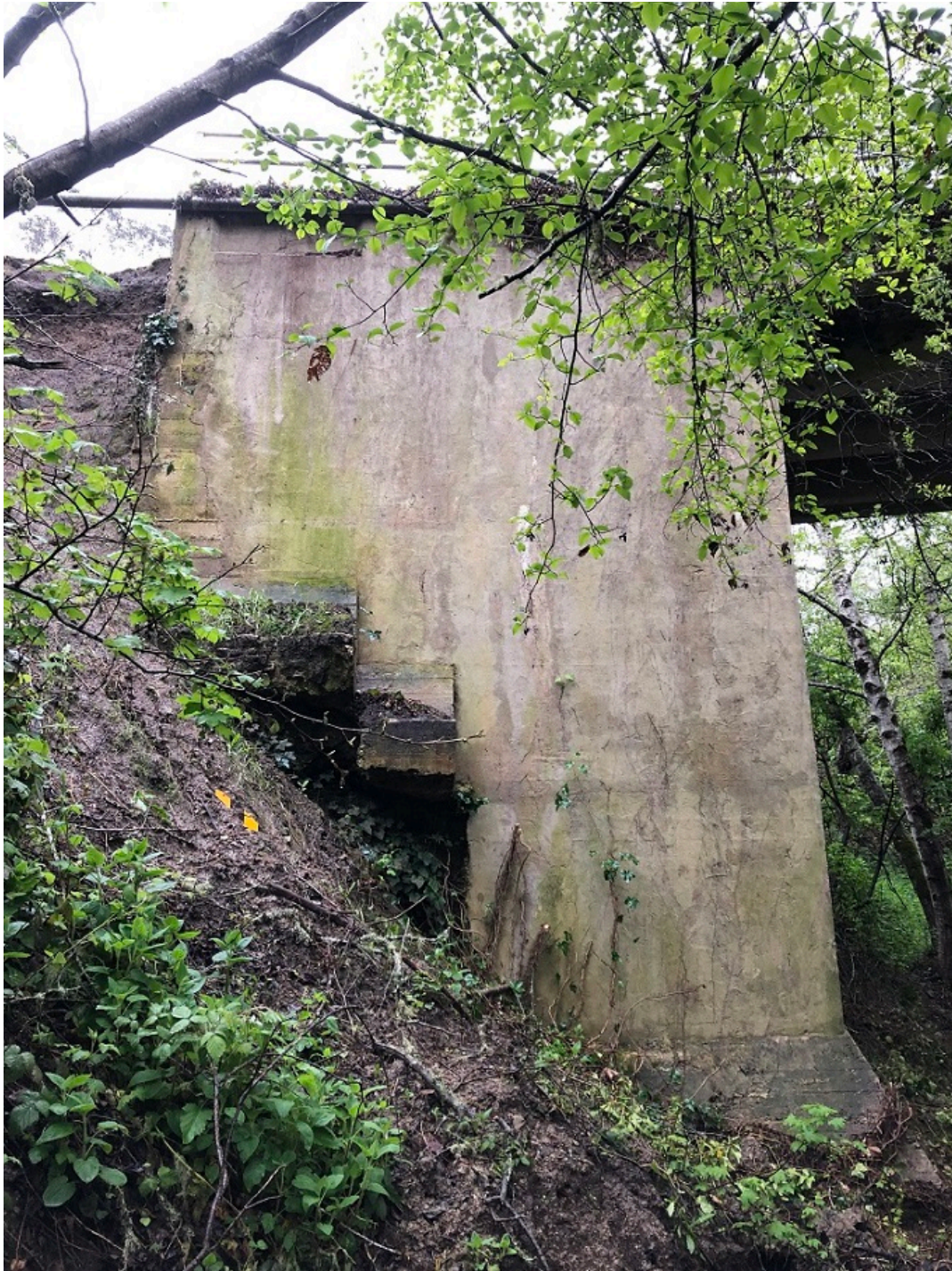
View of the southeast wingwall looking west.
