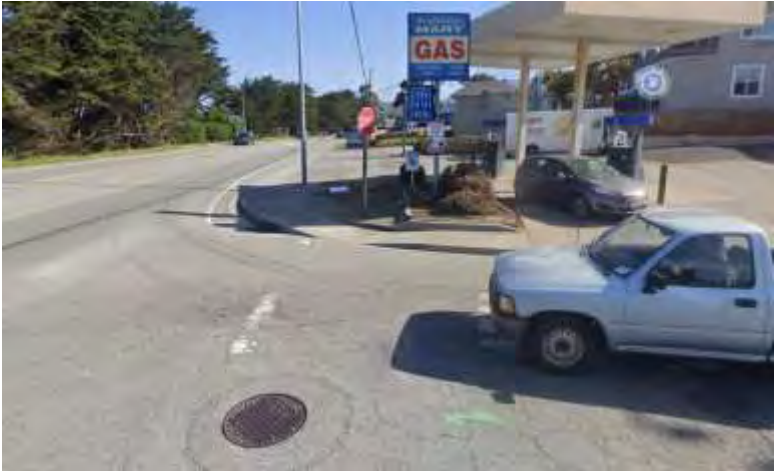
Example of a minor and stop-controlled intersection at Highway 1 and 8 th Street in Montara; 8 th street is the “minor and stop-
