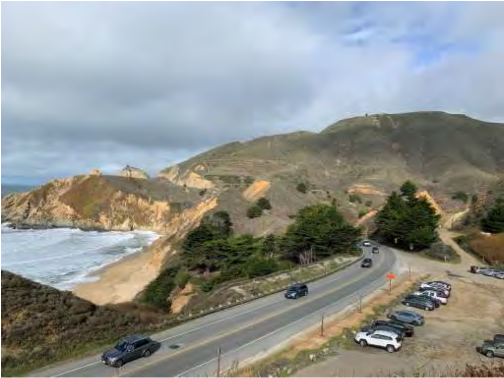
Parking lot with no marked crossing of Highway 1 to reach Gray Whale Cove
