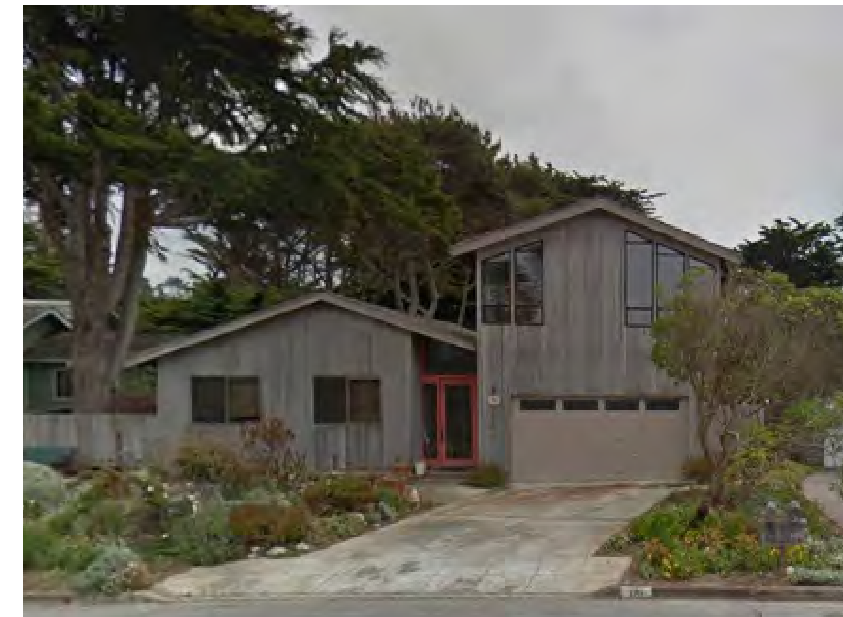
181 ARBOR LANE - EXISTING ADJACENT HOUSE ON THE SOUTH SIDE
