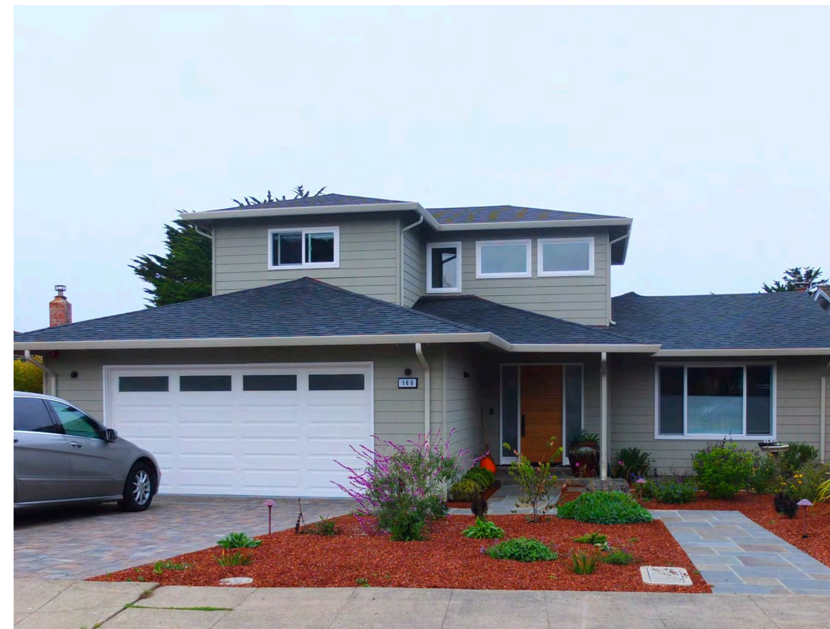
EXISTING ADJACENT HOUSE ON THE NORTH SIDE
