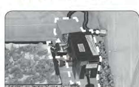
Fig. 19-4 Keep pilot, valve, & shield(s) clear
