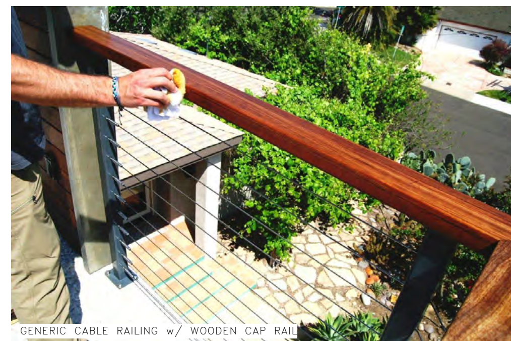
GENERIC CABLE RAILING w/ WOODEN CAP RAIL
