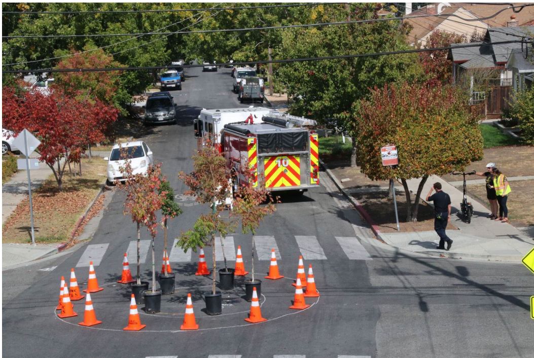
Example of a traffic calming demonstration in the City of Redwood City of a mini-traffic circle - https://www.redwoodcity.org/departments/community-development-department/engineering-transportation/transportation-and-parking/traffic-calming-projects
