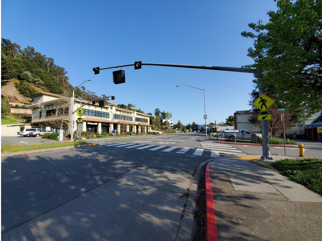
Example of both RRFB and overhead Pedestrian Hybrid Beacon in San Anselmo, California
