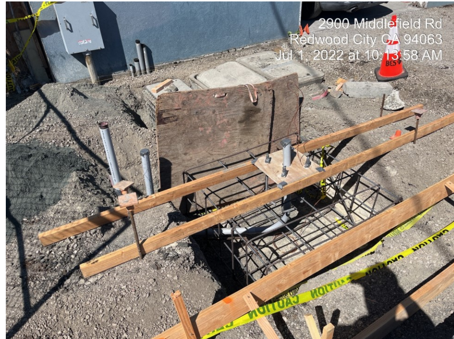
Rapid Rectangular Flash Beacon (RRFB) Foundation
