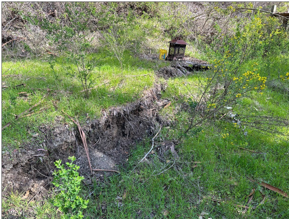
Photo 18: North-facing view of the exposed northwestern extent of the main landslide scarp on the private property at 2175 Higgins Canyon Road. Photo was taken during our last site visit on March 20 th , 2023.
