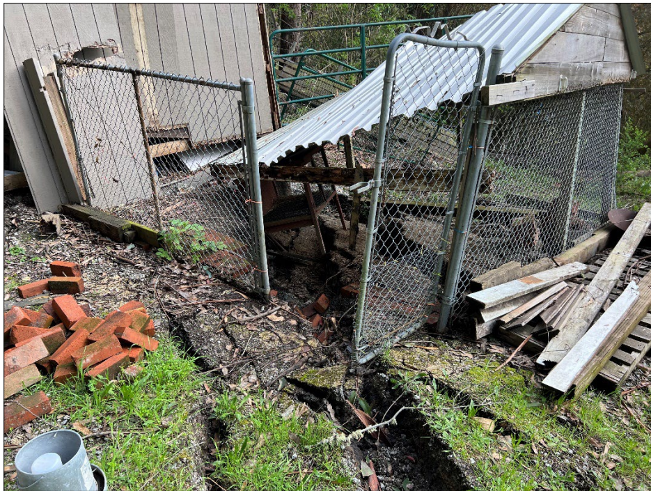
Photo 14: Southeast-facing view of tension cracks on the upslope private property at (2175 Higgins Canyon Road). Photo was taken during our last site visit on March 20 th , 2023.
