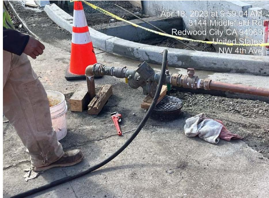
*Cal Water pressure testing after installation
