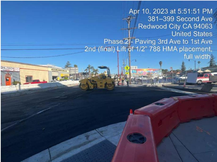
*Drum roller compacting paving*
