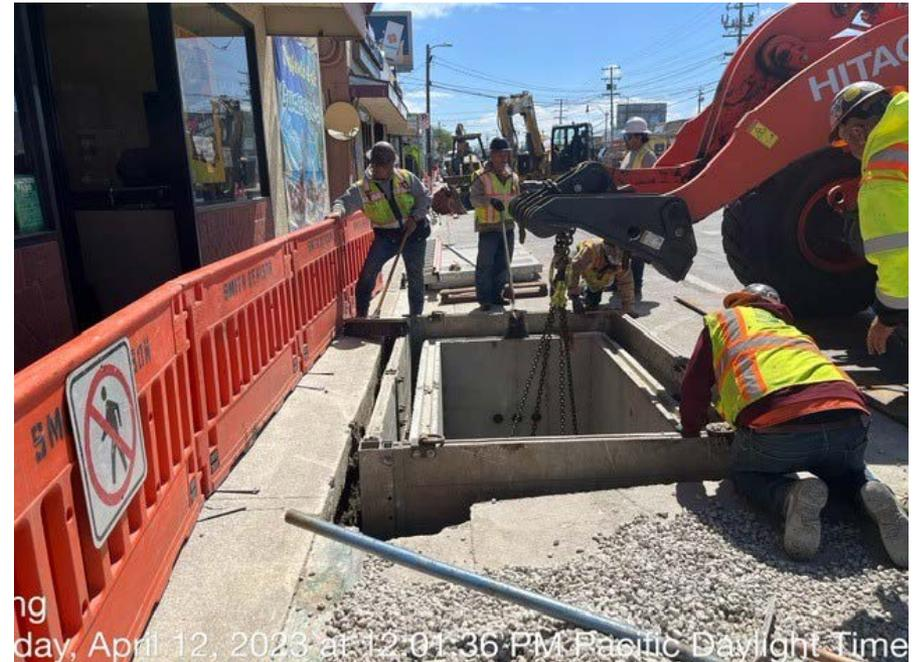
*Installation of new PG&E utility underground vault*
