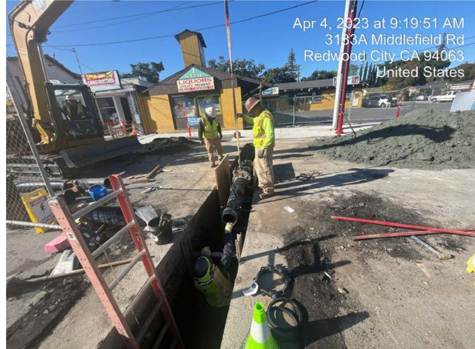
*Waterline wrapped prior to installation*
