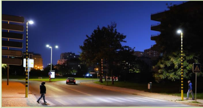
Sidewalk and crosswalk lighting
