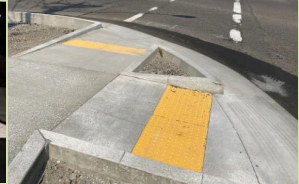
Accessible curb ramps
