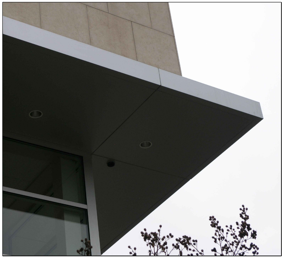
8 ALUM. METAL CLAD CANOPY @ FRONT ENTRANCE
