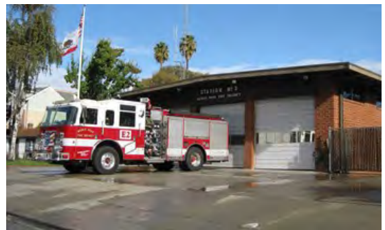
New Menlo Park Fire District Station 2 on University Ave.
