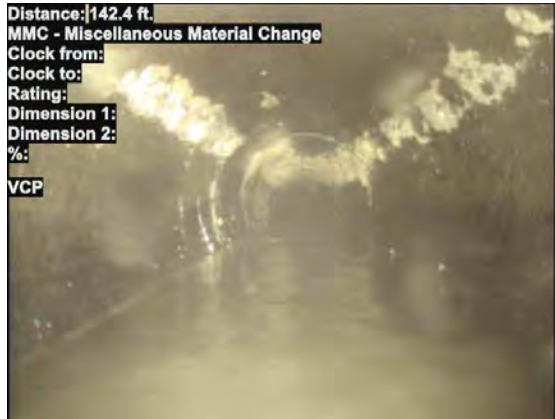
19, 00:14:52, 142.40ft Miscellaneous Material Change / VCP
