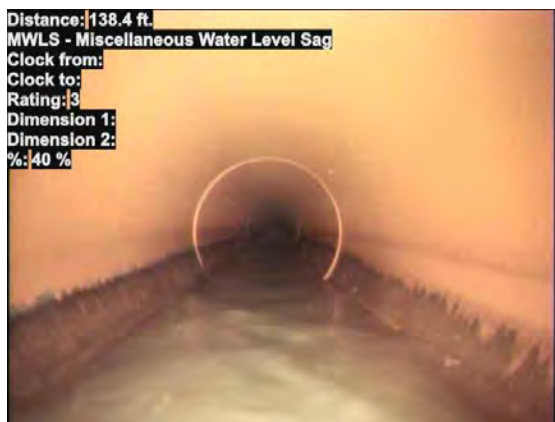
17, 00:08:08, 138.40ft Miscellaneous Water Level, Sag, 40% of the vertical dimension, Finish
