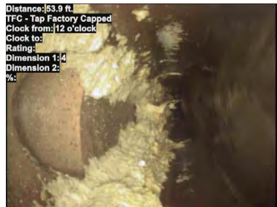
10, 00:06:36, 53.90ft Tap Factory Made Capped at 12 o'clock, dia/height: 4.000inch, within 8 inch
