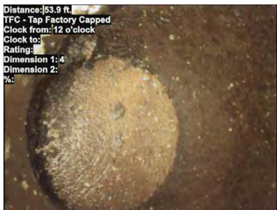
11, 00:06:36, 53.90ft Tap Factory Made Capped at 12 o'clock, dia/height: 4.000inch, within 8 inch
