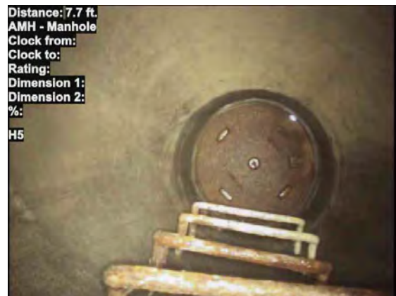
4, 00:01:09, 7.70ft Manhole / H5
