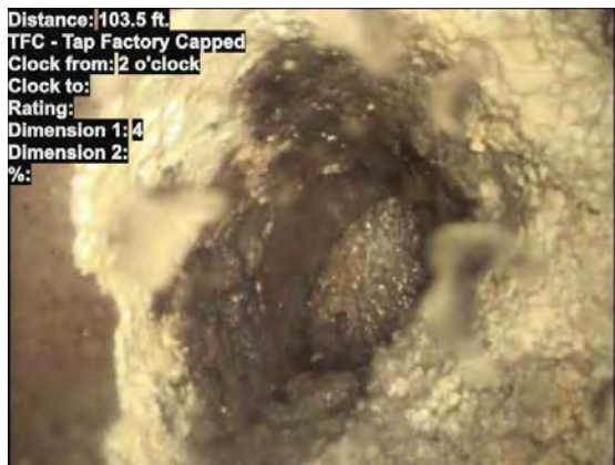
15, 00:13:04, 103.50ft Tap Factory Made Capped at 2 o'clock, dia/height: 4.000inch, within 8 inch
