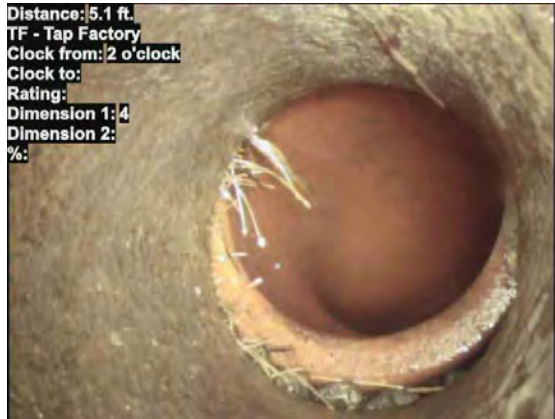
7, 00:02:33, 5.10ft Tap Factory Made Defective at 2 o'clock, dia/height: 4.000inch, within 8 inch / Light Roots
