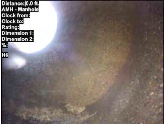
1, , 0.00ft Manhole / H6
