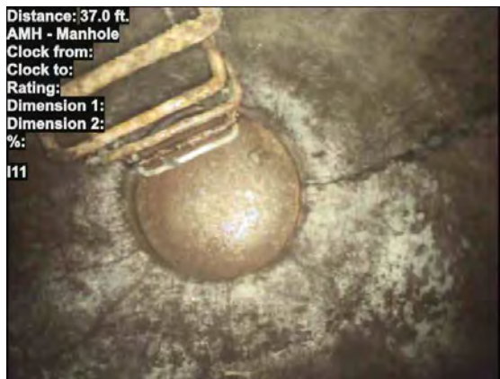
5, 00:02:23, 37.00ft Manhole / I11
