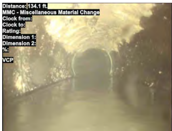
17, 00:14:12, 134.10ft Miscellaneous Material Change / VCP
