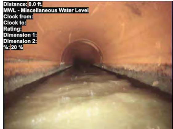
2, , 0.00ft Water Level, 20% of the vertical dimension
