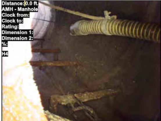
1, , 0.00ft Manhole / H4
