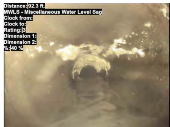
12, 00:12:07, 92.30ft Miscellaneous Water Level, Sag, 40% of the vertical dimension, Finish
