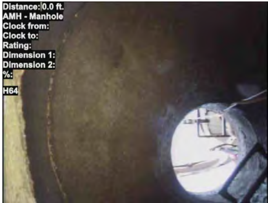
1, , 0.00ft Manhole / H64
