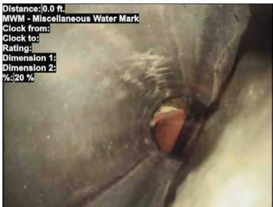
3, 00:00:32, 0.00ft Miscellaneous Water Mark, 20% of the vertical dimension
