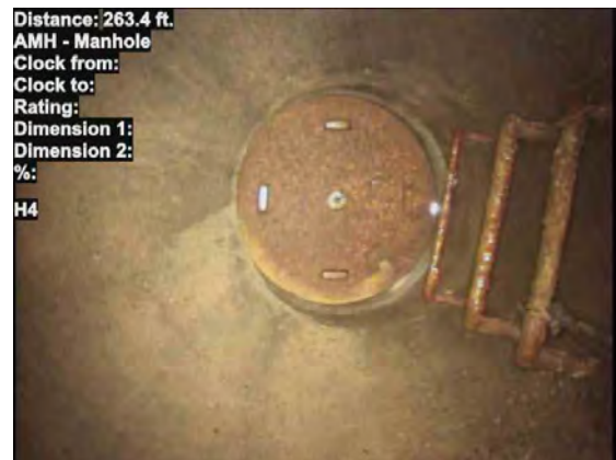
34, 00:16:05, 263.40ft Manhole / H4
