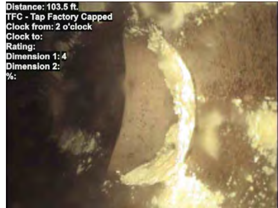
14, 00:13:04, 103.50ft Tap Factory Made Capped at 2 o'clock, dia/height: 4.000inch, within 8 inch
