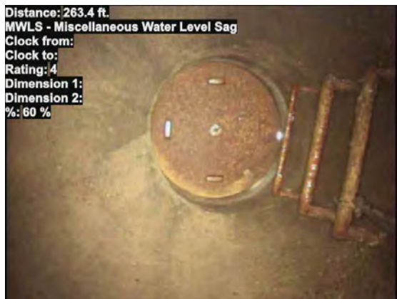
33, 00:15:58, 263.40ft Miscellaneous Water Level, Sag, 60% of the vertical dimension, Finish
