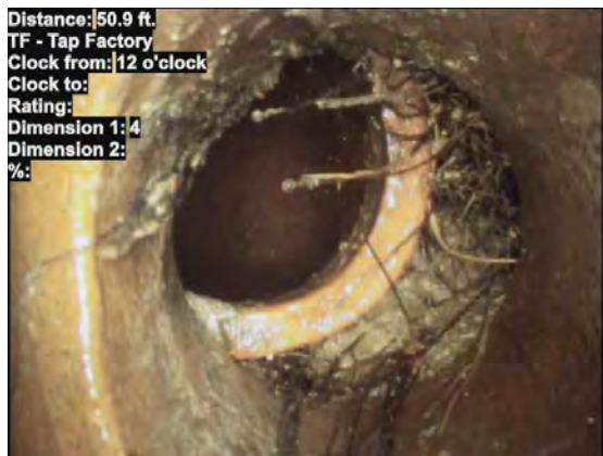
9, 00:05:47, 50.90ft Tap Factory Made Defective at 12 o'clock, dia/height: 4.000inch, within 8 inch / Light Roots
