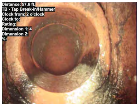
9, 00:04:01, 57.60ft Tap Break-in/Hammer at 2 o'clock, dia/height: 4.000inch, within 8 inch
