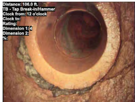
12, 00:05:44, 106.00ft Tap Break-in/Hammer at 12 o'clock, dia/height: 4.000inch, within 8 inch
