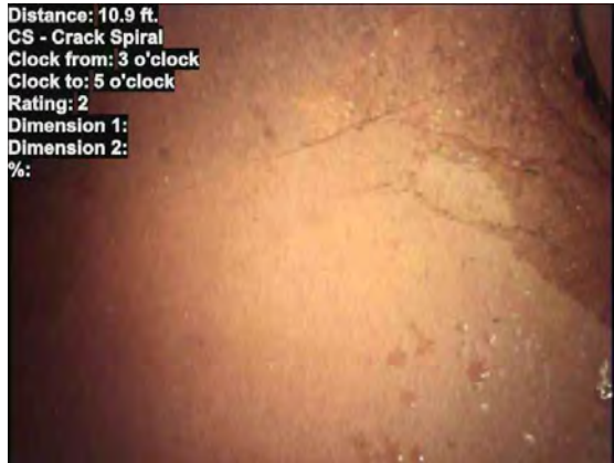
7, 00:01:46, 10.90ft Crack Spiral from 3 o'clock to 5 o'clock
