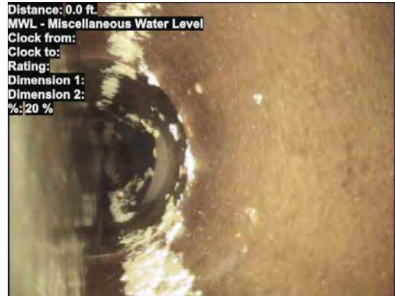
2, , 0.00ft Water Level, 20% of the vertical dimension
