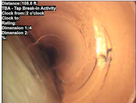
13, 00:06:21, 108.60ft Tap Break-in Activity at 2 o'clock, dia/height: 4.000inch, within 8 inch
