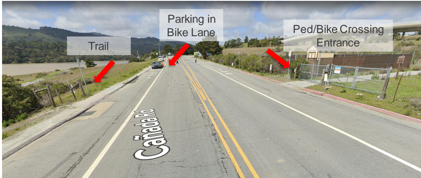
Existing Conditions (looking north)
