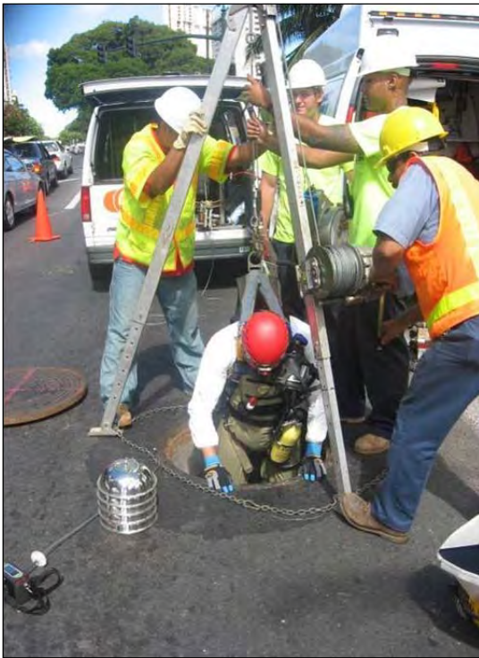
Photo 1. Confined Space Entry
