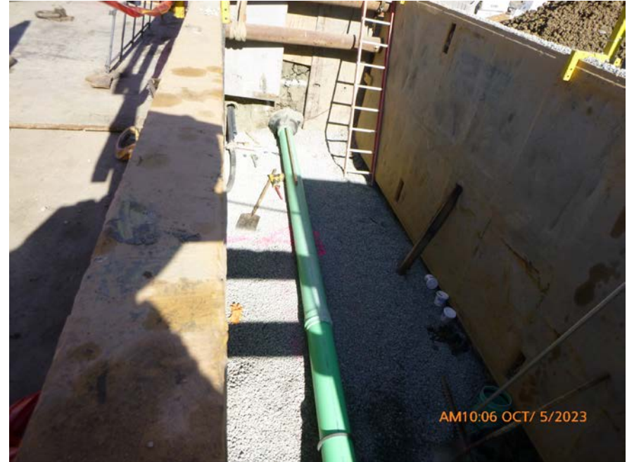
Sewer pipe installed and connected at the receiving pit
