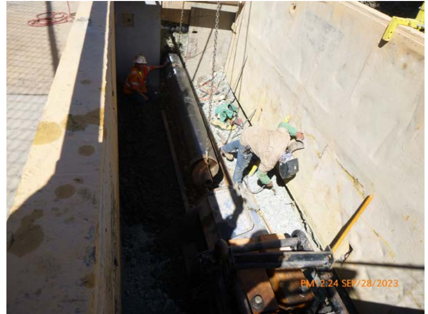
Jack and Bore Casing being installed
