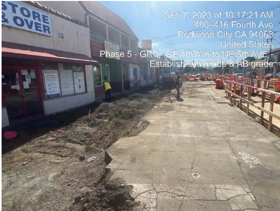
Phase 5 sidewalk removed
