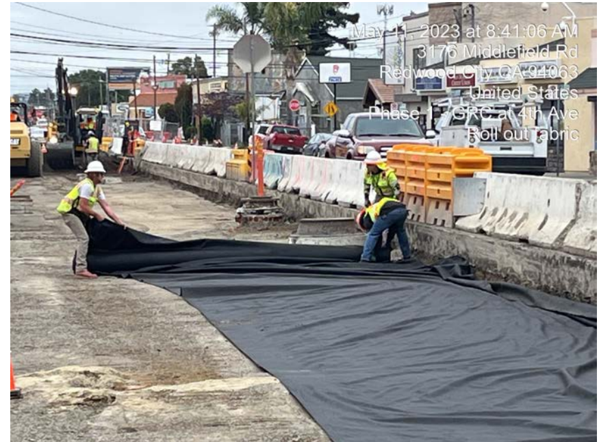
Phase 1 Roadway work
