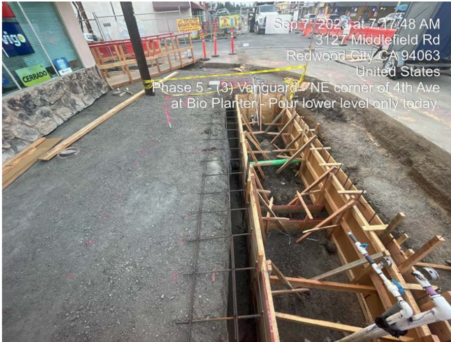
Phase 5 sidewalk formwork
