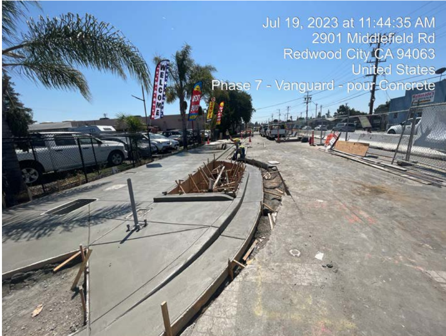
Phase 7 concrete work completed
