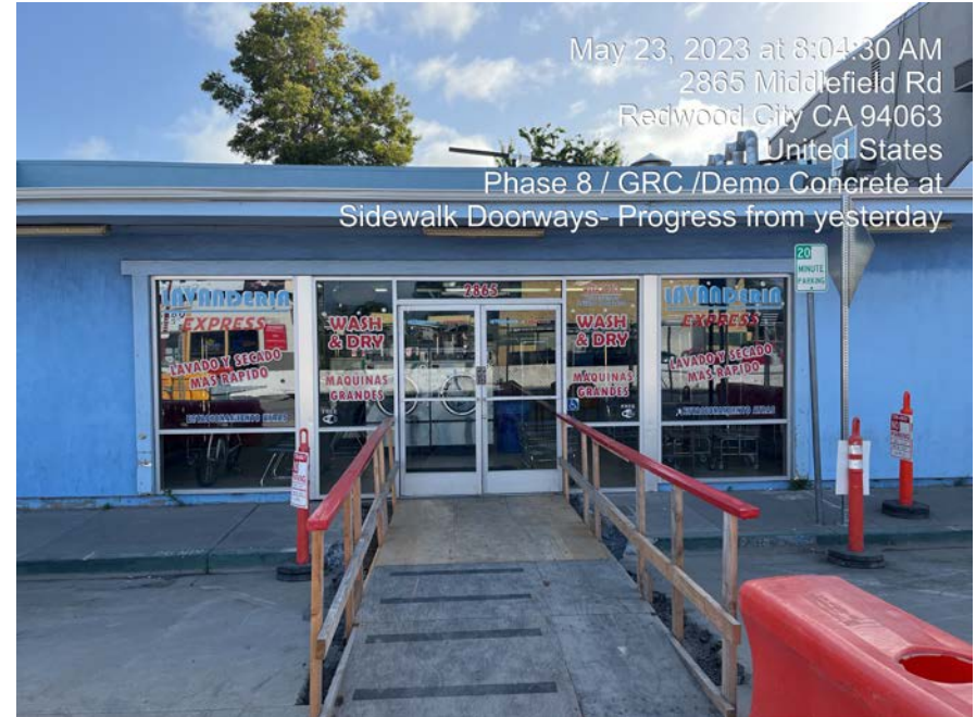
Public Convenience – Temporary Business Access
