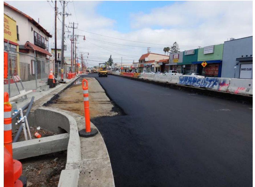
Phase 1 Roadway Paving
