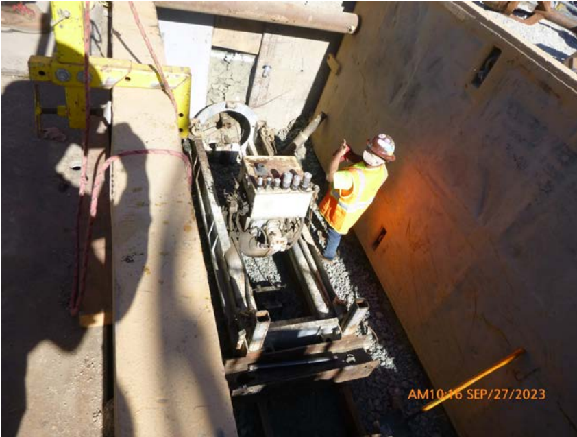
Jack and Bore pilot hole being installed
