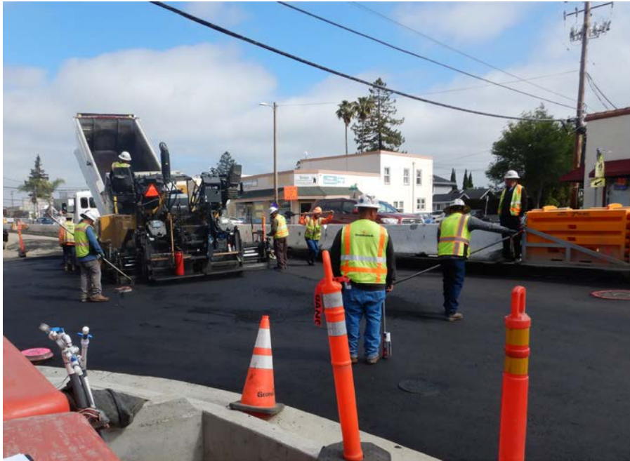
Phase 1 Roadway paving
