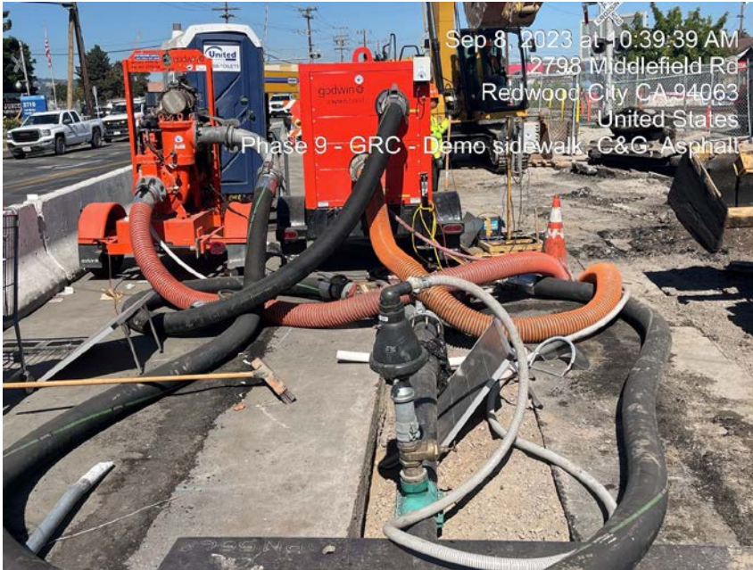
Temporary Sewer by-pass system
