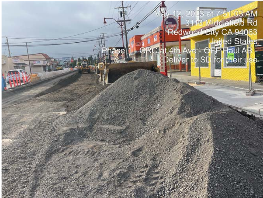
Phase 1 Roadway work
