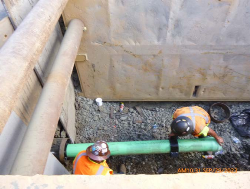
Sewer pipe being installed thru casing
