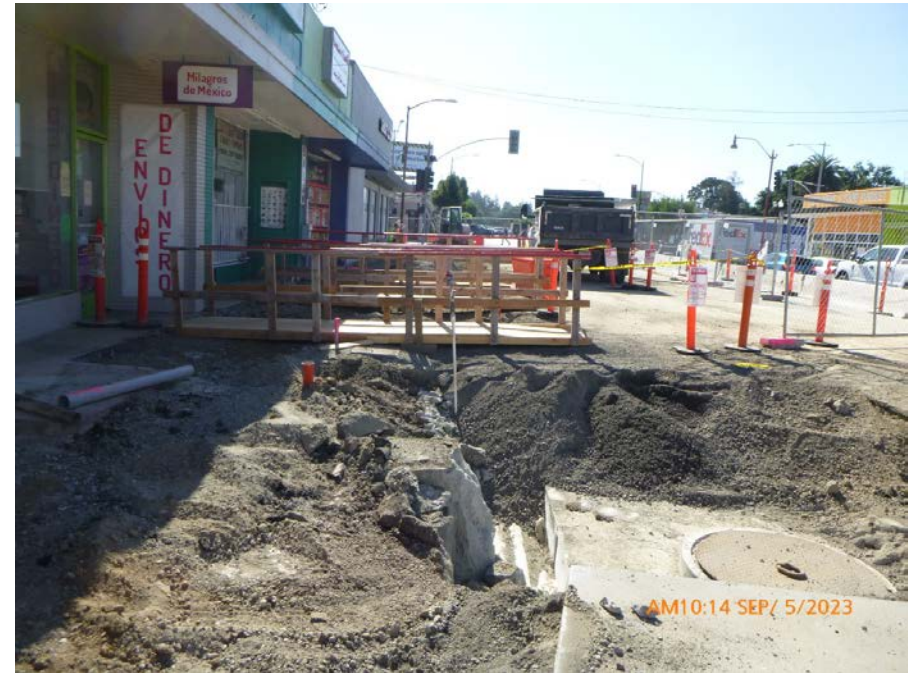
Phase 5 sidewalk removed
