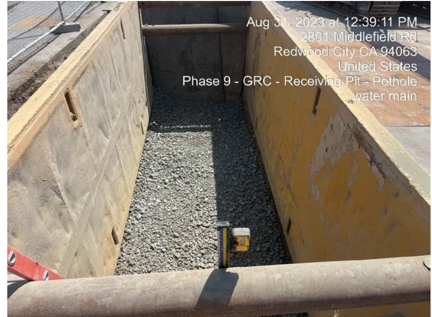
Jack and Bore Entry Pit
