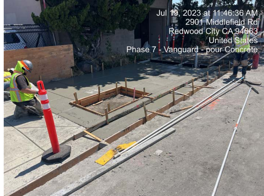
Phase 7 concrete work completed
