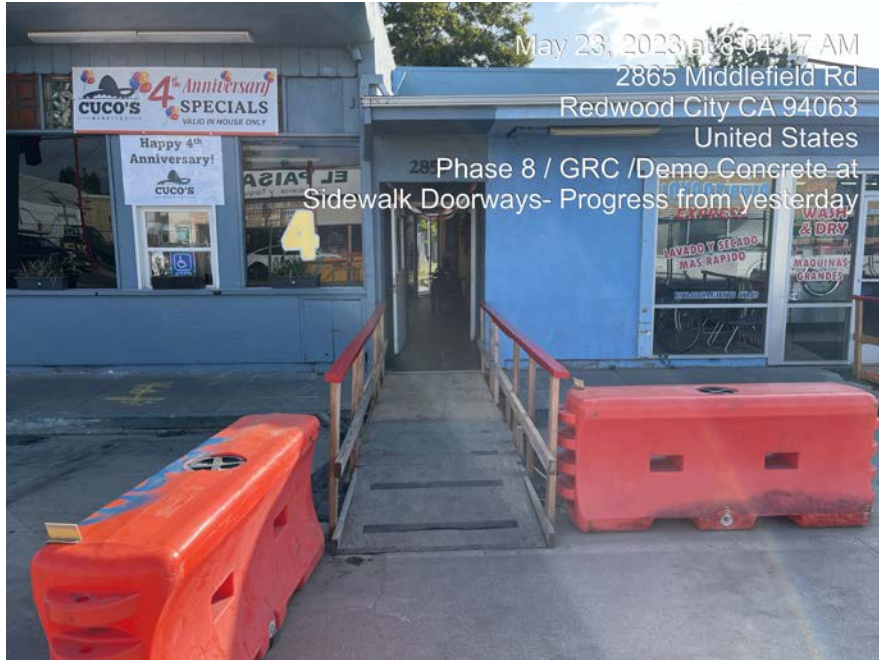
Public Convenience – Temporary Business Access
