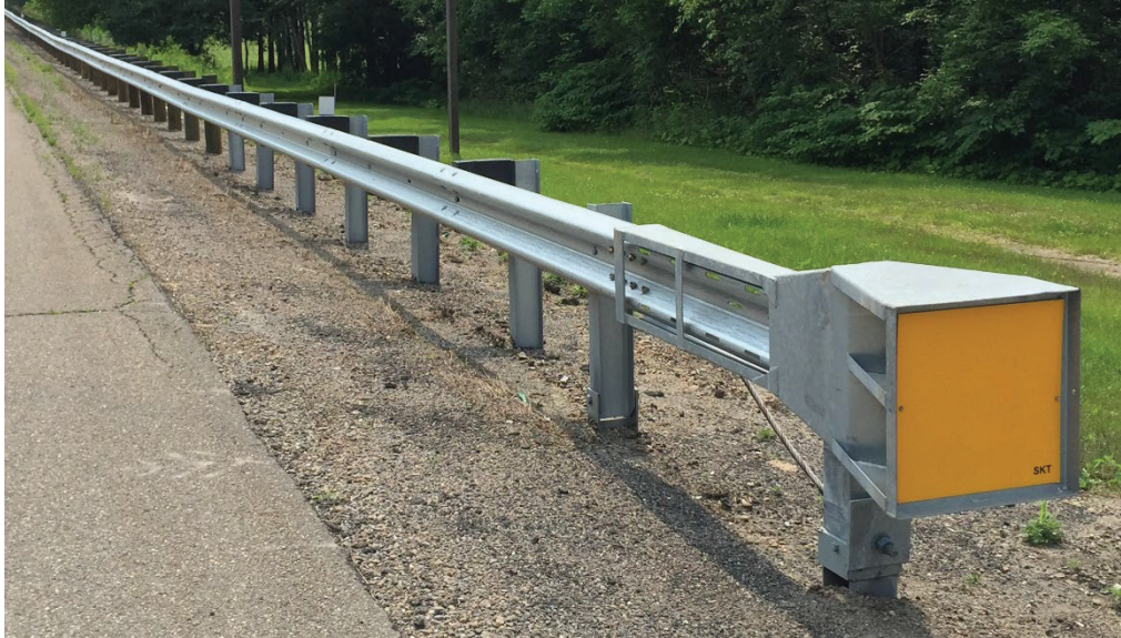
Figure 3: Example Midwest Guardrail System with crash cushion
