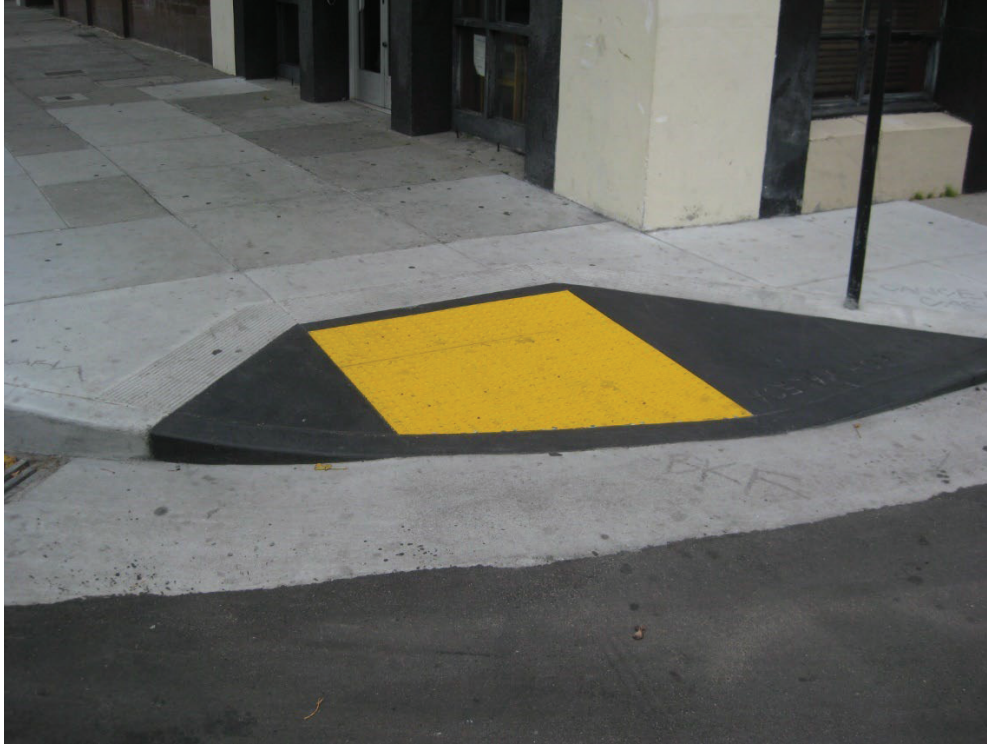
Figure 5: Example ADA-compliant curb ramp
