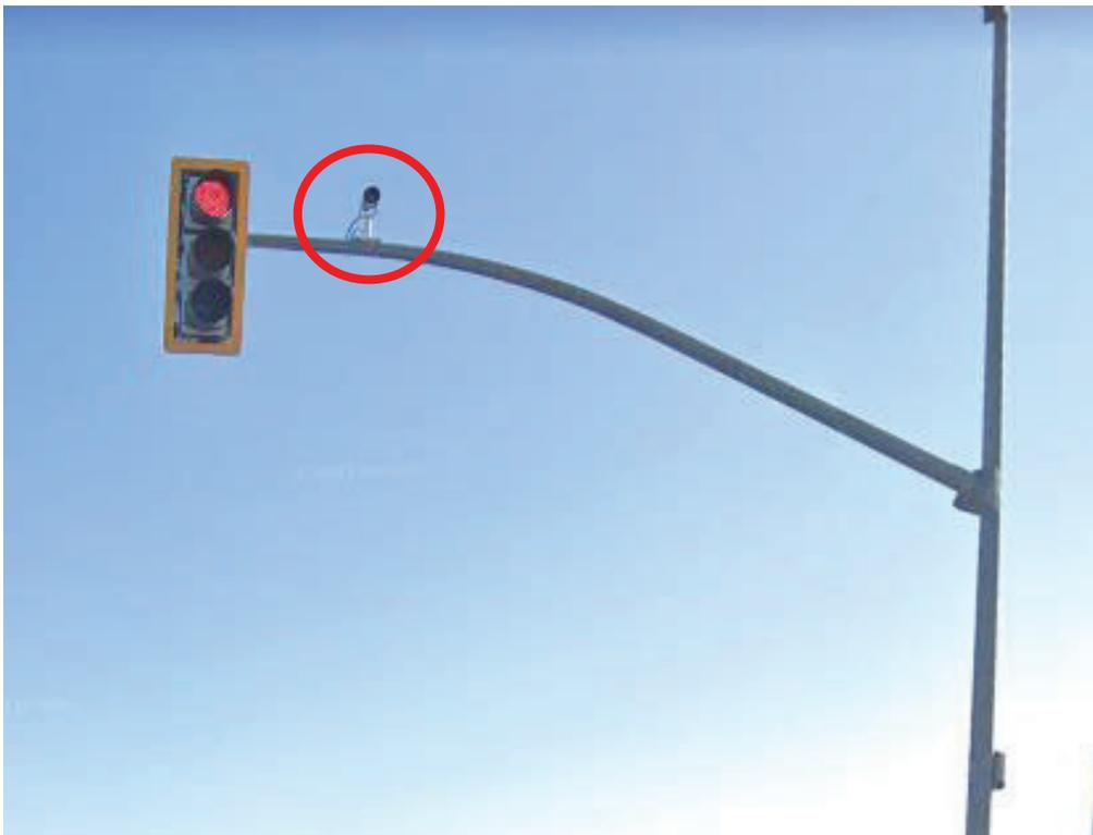
**Figure 4: Example fixed intersection camera/CCTV**
