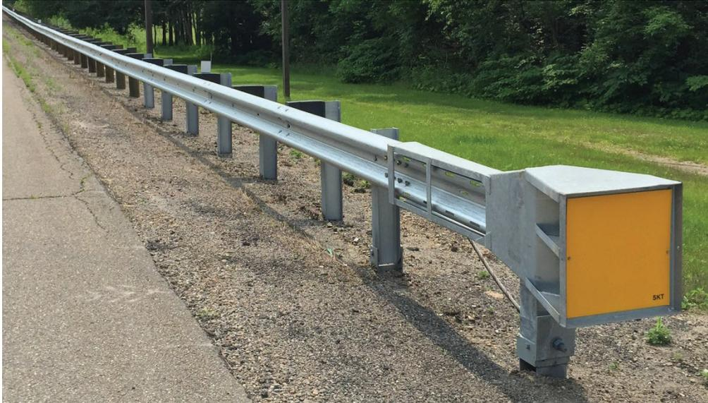
**Figure 3: Example Midwest Guardrail System with crash cushion**
