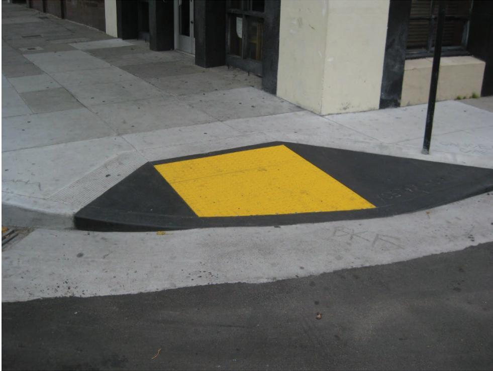
**Figure 5: Example ADA-compliant curb ramp**
