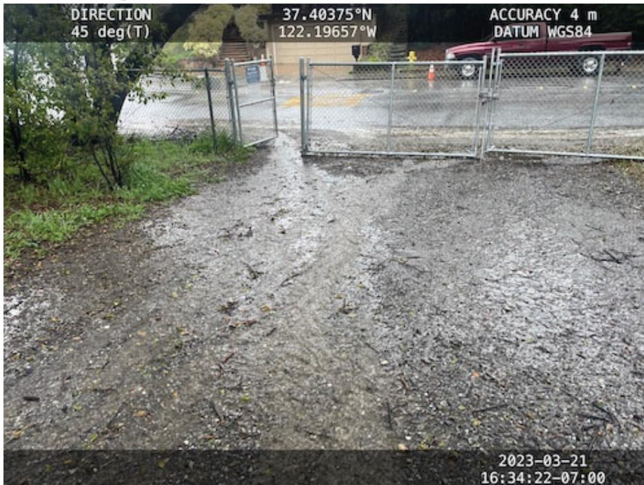
Channelized water from fire access road overwhelming the storm drain
