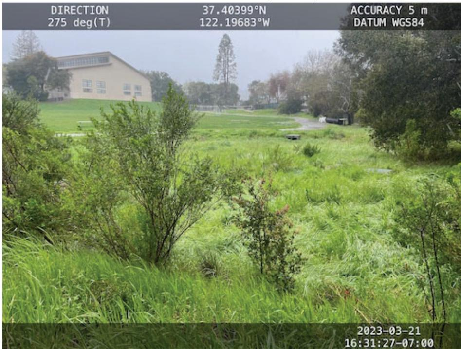
Close up of retention basin showing no retained water despite channelized water overwhelming storm drain only 75 feet away
