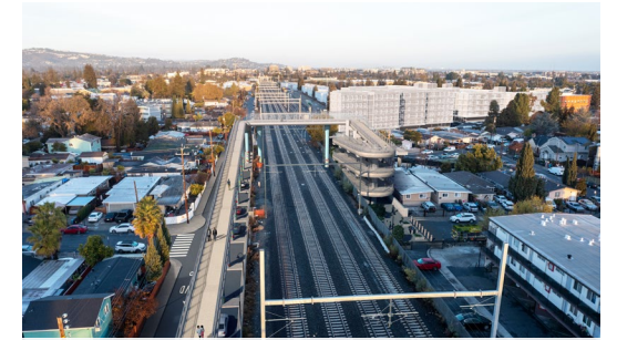
Aerial view of bridge facing west
