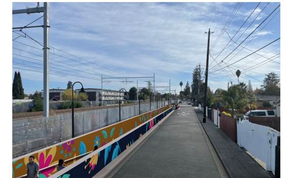
Westmoreland Avenue entrance to tunnel with art along ramp walls
