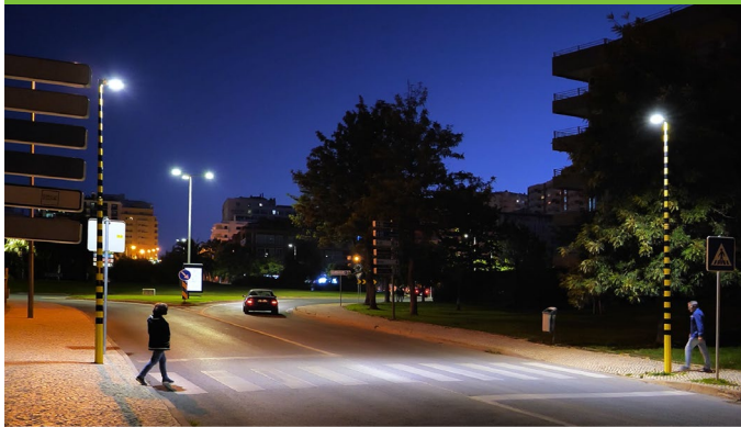
Sidewalk & Crosswalk Lighting
