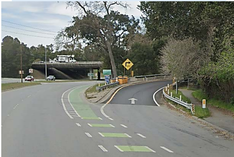
Bike/Trail Crossing at SB On-Ramp
