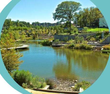
Surface detention basins
