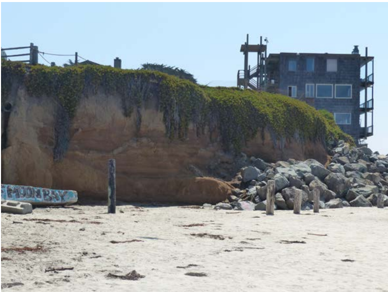
Photo 2. Soil Nail Wall 2 Installation Location Southwest of Pedestrian Bridge.
