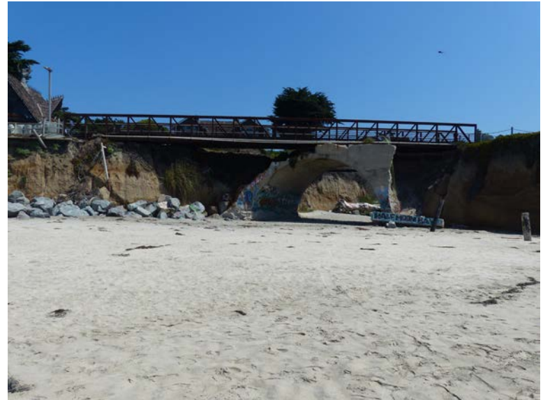
Photo 7. Existing Pedestrian Bridge.
