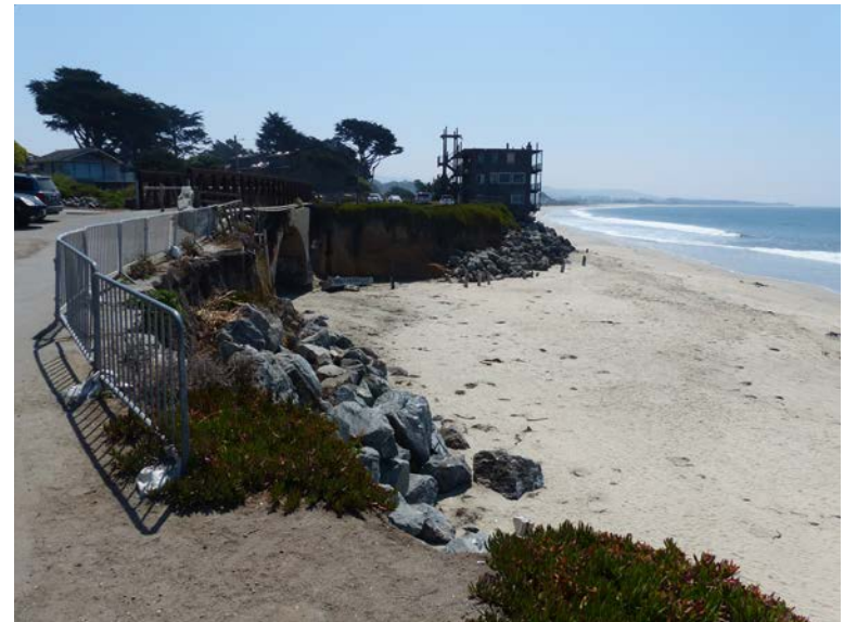
Photo 8. Existing Rock Slope Protection.
