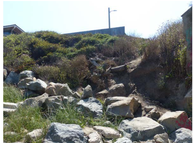
Photo 4. Location of Proposed Access Southeast of Pedestrian Bridge.
