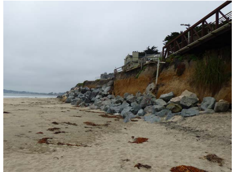
Photo 3. Soil Nail Wall 3 Installation Location Northeast of Pedestrian Bridge.
