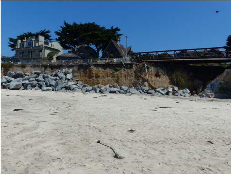
Photo 1. Soil Nail Wall 1 Installation Location Northwest of Pedestrian Bridge.
