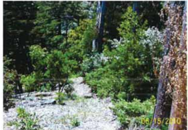
Figure 12. Fey Drive. Sewer line runs through a wooded area upslope of Fey Drive between residences. Shrubs and overhanging trees may provide bird nesting habitat.
