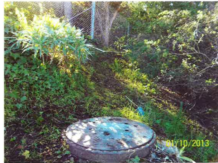
Photo 8. Typical view of easement areas for Adeline Drive.
