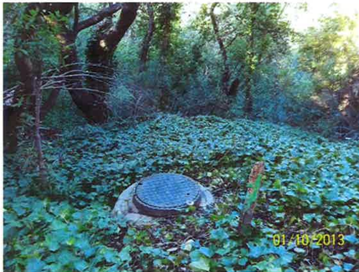
Photo 7. Typical view of easement areas for Adeline Drive.
