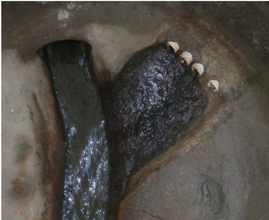
Figure 1-9. Drain Pipes Connected at Manhole 67
