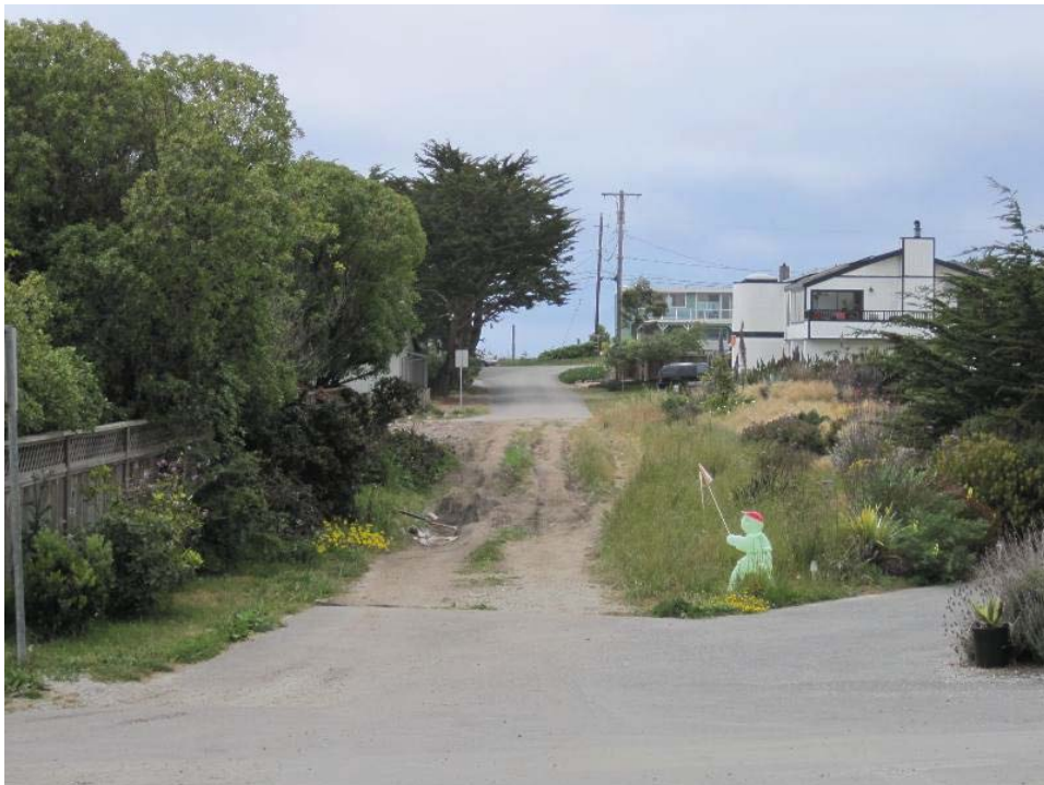
Photo 4: View of Del Mar Avenue facing northwest from Precita Avenue (May 2013).
