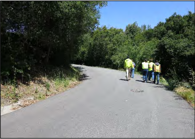
Photo 18. Example of a paved ditch along Occidental Way in the Emerald Hills neighborhood. (May 2015)
