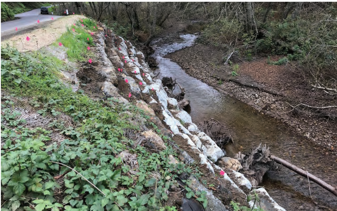
Photo 4. Completed bank stabilization site along Gazos Creek and Gazos Creek Road.
