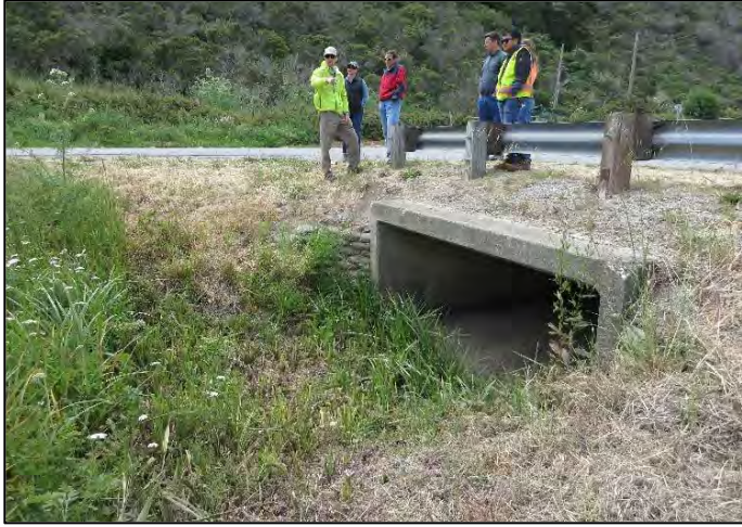
Photo 9. Concrete box culvert at Cloverdale Road and Butano Cutoff Road in Pescadero. Potential need for sediment and vegetation removal in the future. (May 2015)
