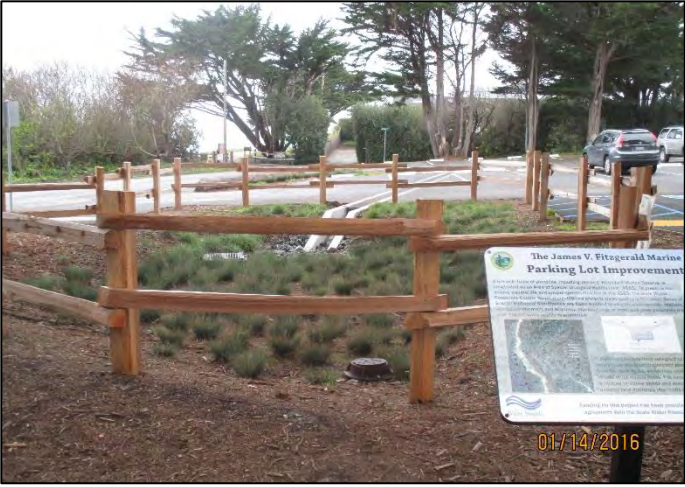
Photo 12. Bioretention swale at the Fitzgerald Marine Reserve parking lot, which requires periodic vegetation removal, light sediment clearing and revegetation. (January 2016)
