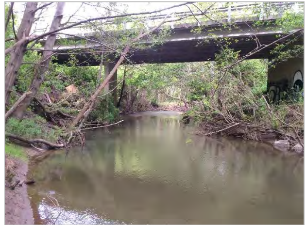
Photo 1. Upstream side of Pescadero Creek Road bridge near Cloverdale Road. (April 6, 2017)
