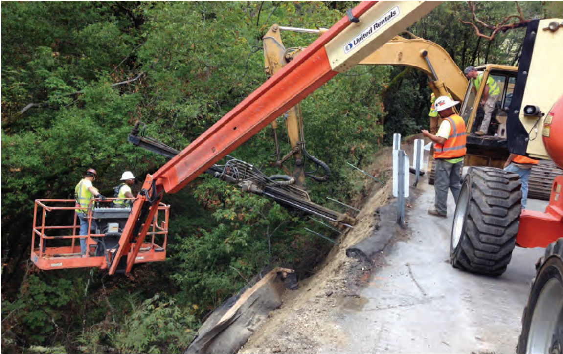
Photo 5. Example of soil nailing at a bank stabilization site along Alpine Road. (September 2014)
