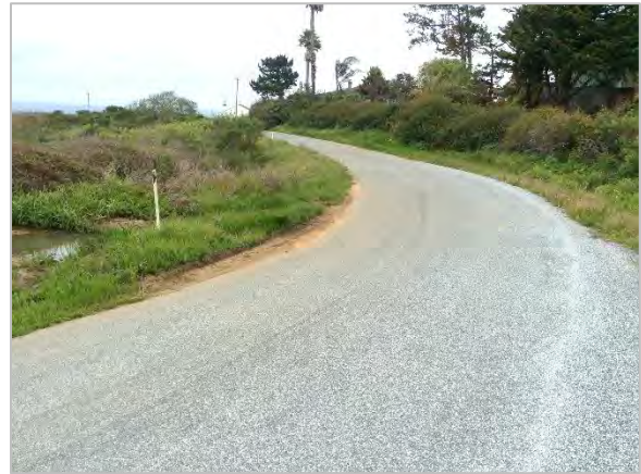
Photo 1. Pigeon Point Road at Mile 0.4 culvert. (April 6, 2017)
