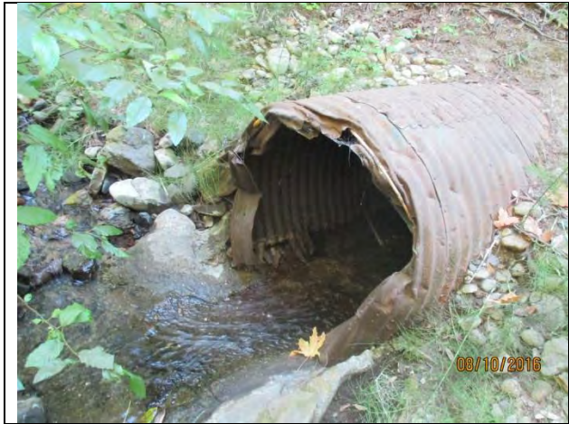
Photo 2. 0.9 Alpine culvert inlet (August 10, 2016).
