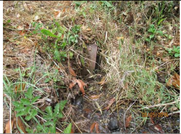
Photo 3. 1.5 Alpine culvert inlet; a seep was observed at the inlet and in the ditch in the vicinity of the culvert (August 2016).
