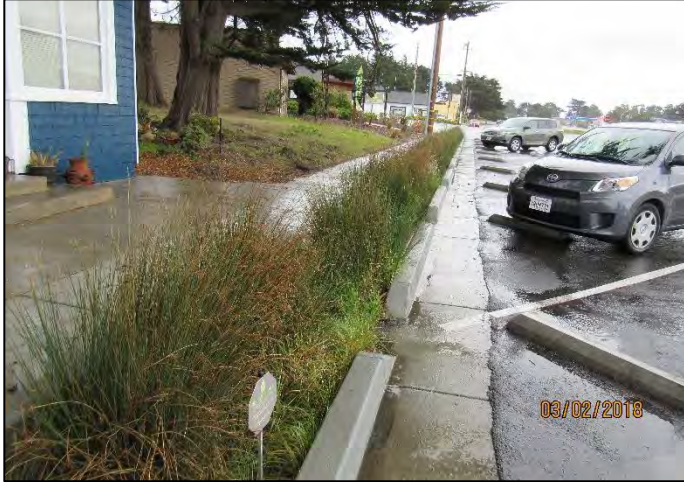
Photo 11. Bioretention swale along Carlos Street in Moss Beach that requires periodic vegetation removal, light sediment clearing, and planting. (March 2018)
