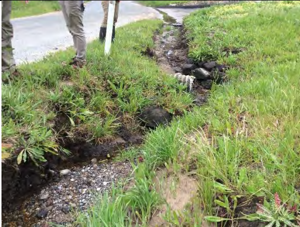
Photo 8. The upstream side of Mile 0.5 culvert. The culvert conveys surface runoff from Pigeon Point Road and a 600-foot (approximate) private driveway (April 6, 2017)
