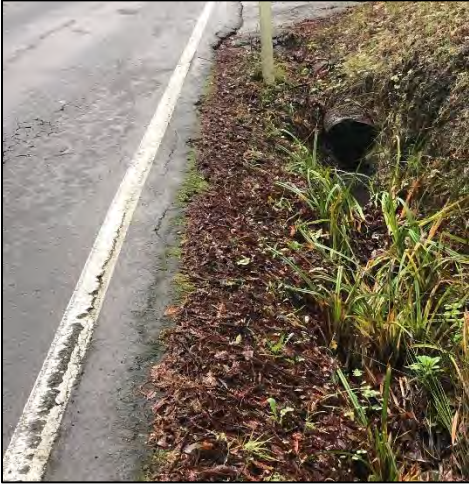
Photo 16. Example of an unpaved ditch and roadside culvert along Pescadero Creek Road and entrance to Sam McDonald Park. (December 2019)
