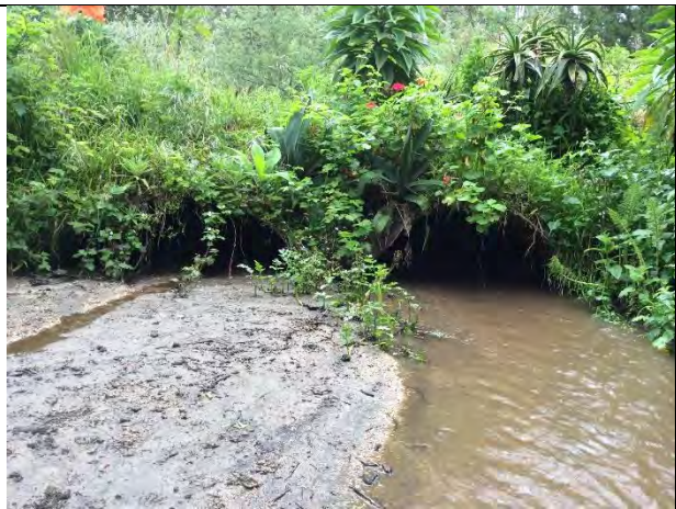
Photo 3. The downstream side of the culverts at Harte Street. (April 6, 2017)
