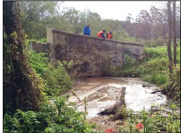
Photo 1. The downstream face of the George Street bridge. (April 6, 2017)
