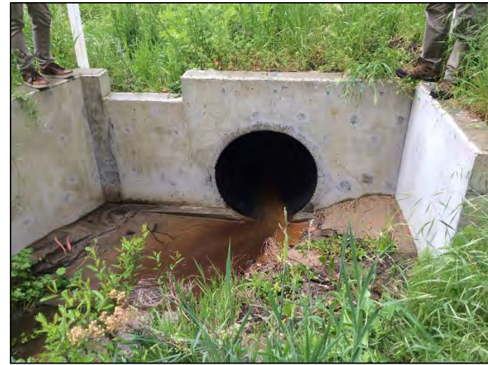
Photo 8. Culvert near George Street bridge that drains to Montara Creek. (April 2017)
