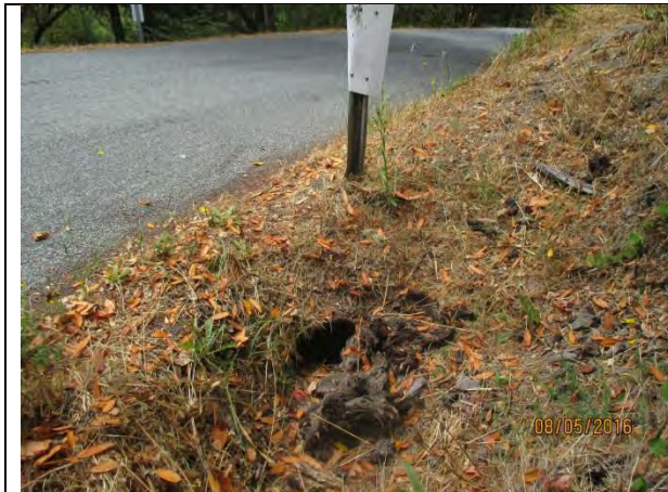
Photo 2. 2.5 Alpine culvert inlet looking southwest (August 5, 2016)
