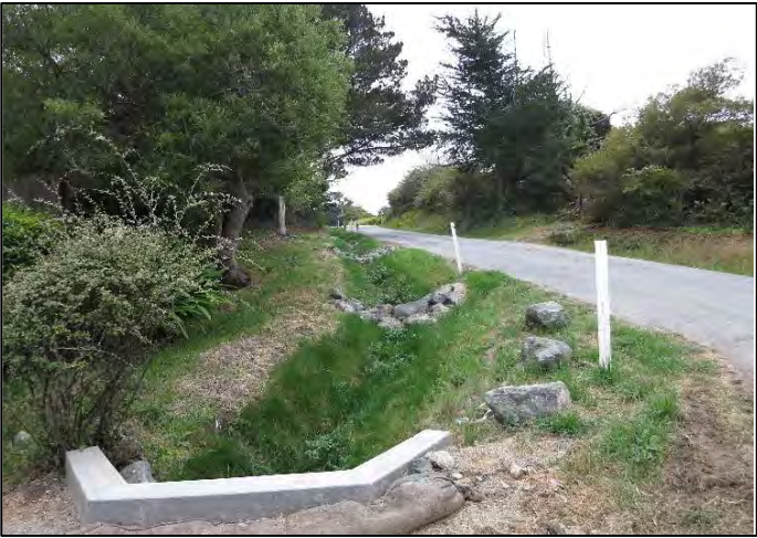
Photo 8. LID enhancements consisting of turf reinforcement mat, native grass sod, and rock check-dams that were recently installed along Farallone Avenue in Montara. (May 2015)
