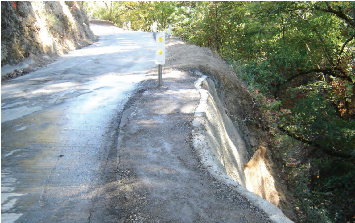
Photo 6. Example of a retaining wall at a bank stabilization site along Alpine Road. (October 2014)
