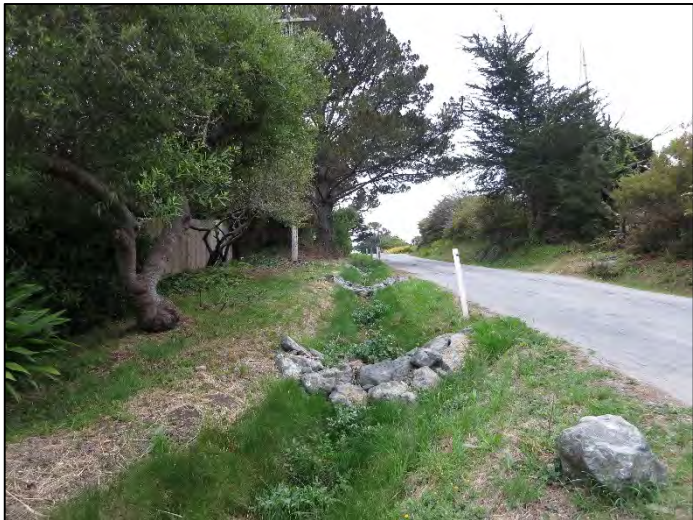
Photo 3. LID ditch along Farallone Avenue in Montara (May 2015)
