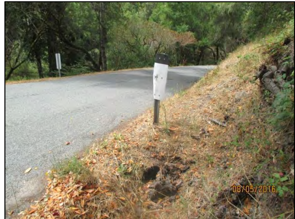
Photo 1. Maintenance work area and Alpine Road looking southwest. (August 5, 2016)
