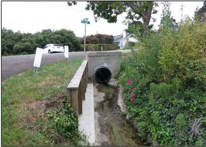
Photo 7. Paved ditch downstream of Farallone Avenue and Kanoff Street in Montara. Ditch is routinely maintained with a Vac-Con truck. (May 2015)
