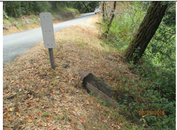
Photo 3. 2.5 Alpine culvert outlet looking northeast (August 5, 2016)
