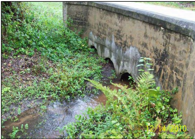
Photo 3. George Street bridge. Sediment and vegetation removal needed in the future. Bridge could also benefit from paint removal. (December 2010)
