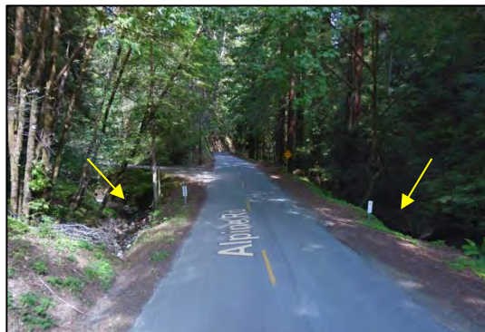
Photo 1. Maintenance work area and Alpine Road looking east towards Heritage Road. Arrow on the left points to culvert inlet for tributary; arrow on the right points to culvert outlet (May 2011).
