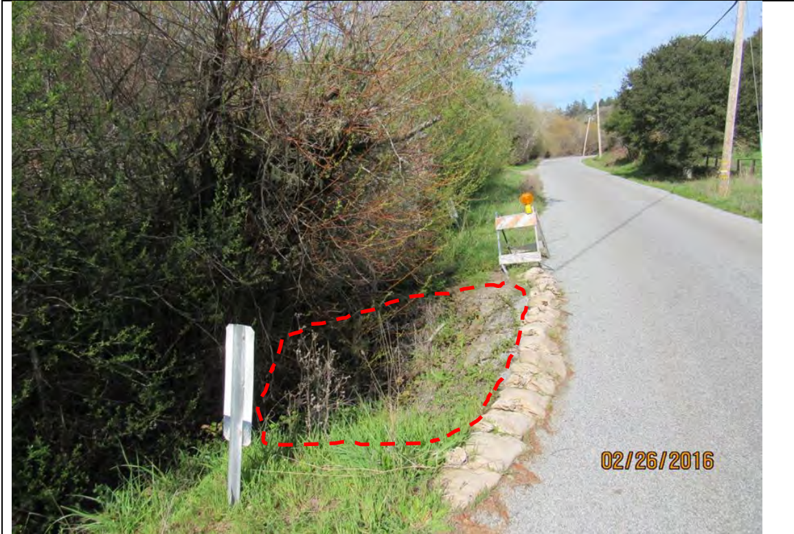
Photo 5- Existing vegetation at slip out location #3, looking north. (February 26, 2016)
