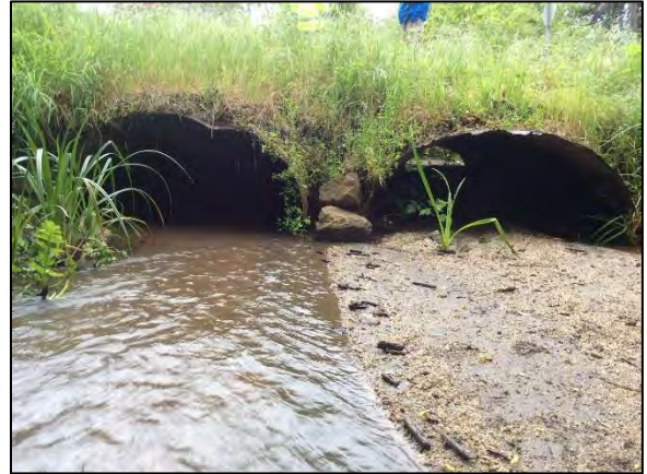
Photo 1. Upstream side of the Harte Street culvert. (April 6, 2017)
