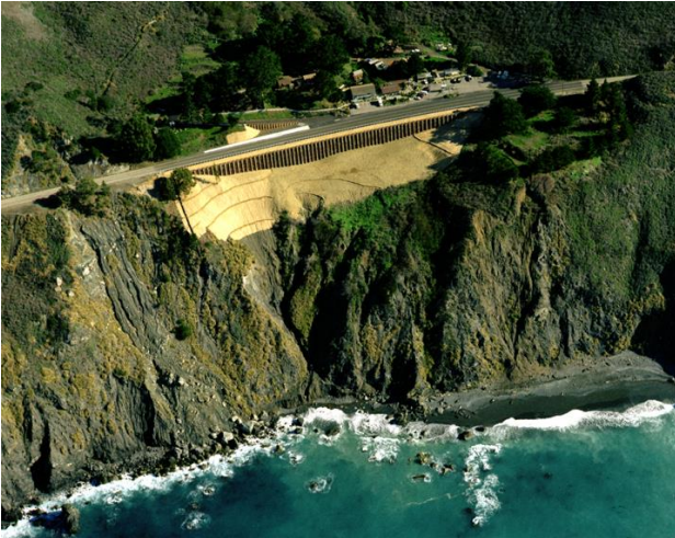
Retaining wall supporting Highway 1 in Monterey County
