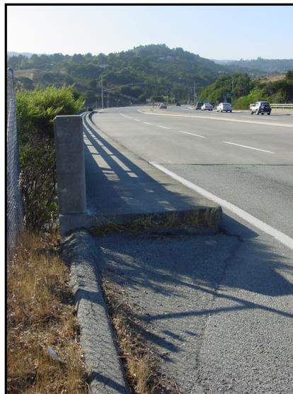
*Sidewalk with no curb ramp on SR92 Overpass, between the signalized study intersections*
