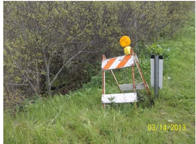
Photo 23 – Photo of traffic barricade directly over sinkhole and culvert disconnection point.
