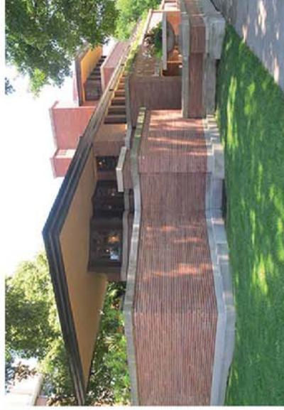
**Roof Pitch:** Roof pitches shall be a maximum 4:12 low-pitched hip roof with deep overhanging eaves, a minimum of 36". Depending on the design a gable might be considered. Roof form should have a strong balanced horizontal element, roof extension or cantilevered projection at the eaves. Roofs often extend over exterior rooms and/or walkways.
