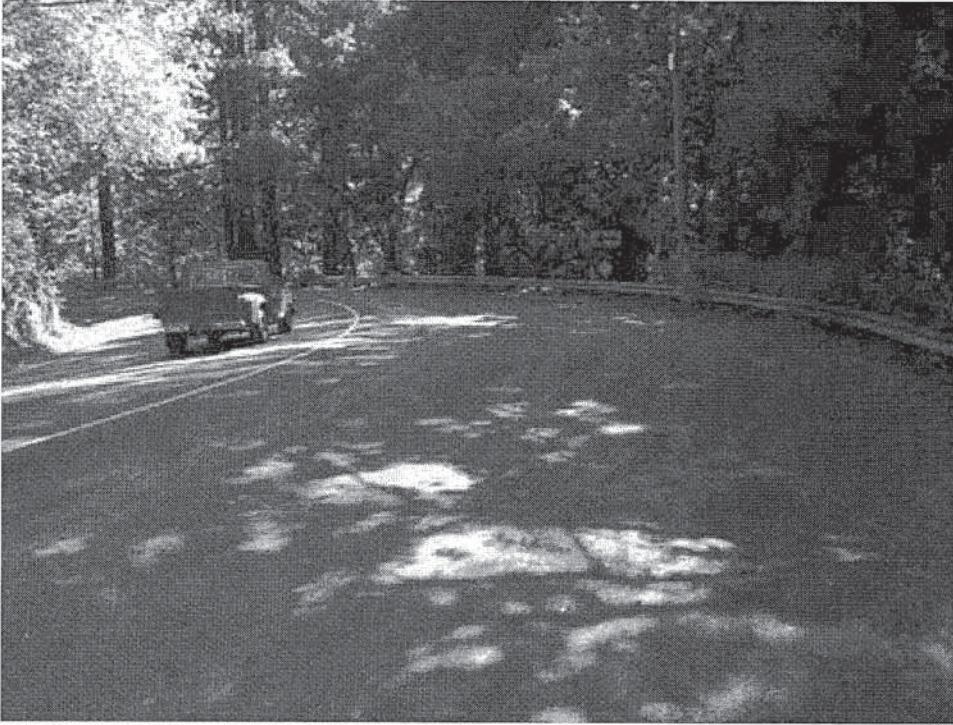
Photo 5: Node 050A Area Overview (South)
