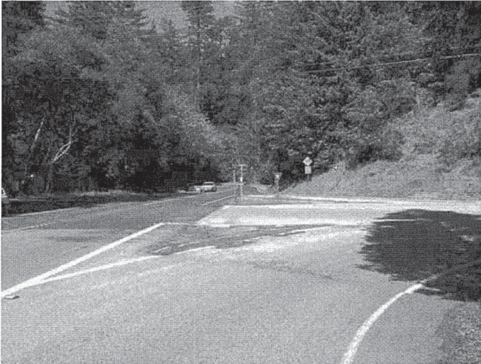
Photo 1: Node 047B Area Overview (North)
