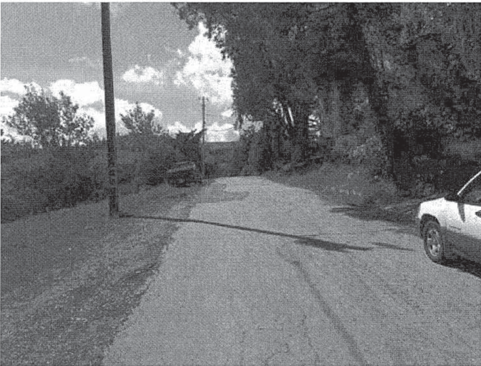
Photo 2: Node 048A Area Overview (West)
