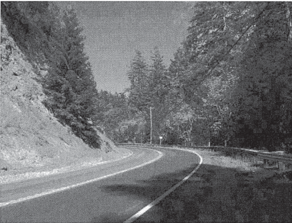
Photo 4: Node 049A Area Overview (East Northeast)
