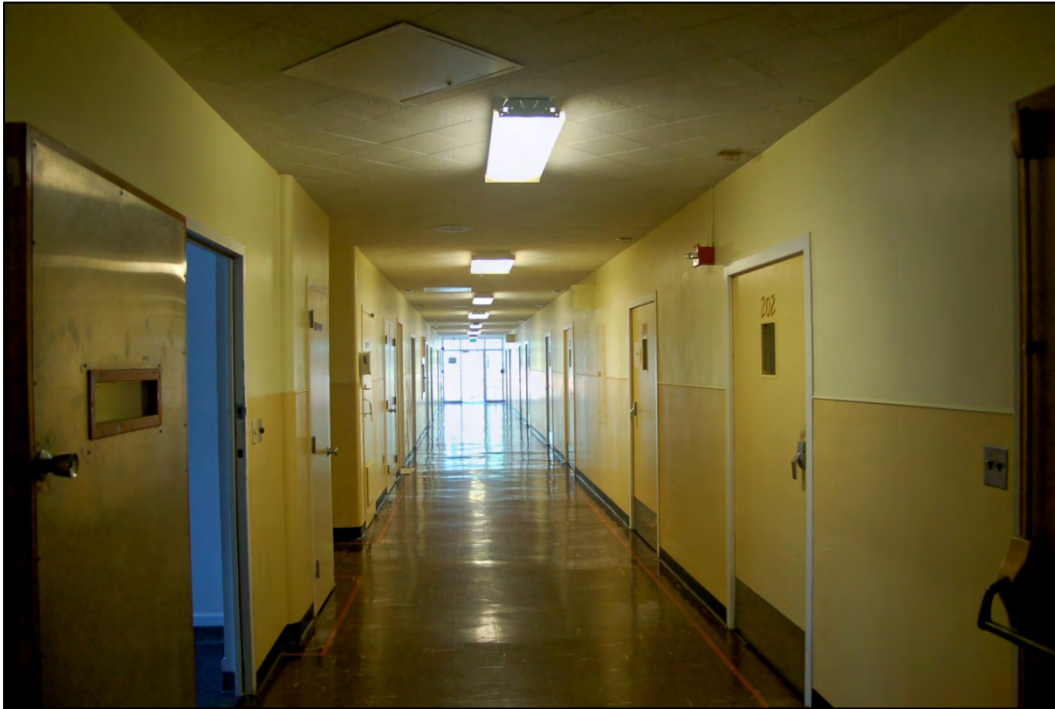
Second floor corridor lined with doors to patient rooms
