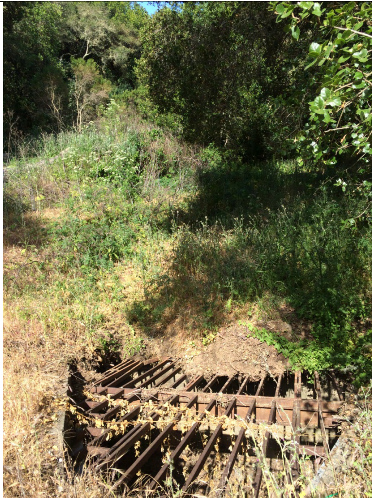
Photo 1: Cordilleras Creek stormdrain inlet upstream of existing development.
