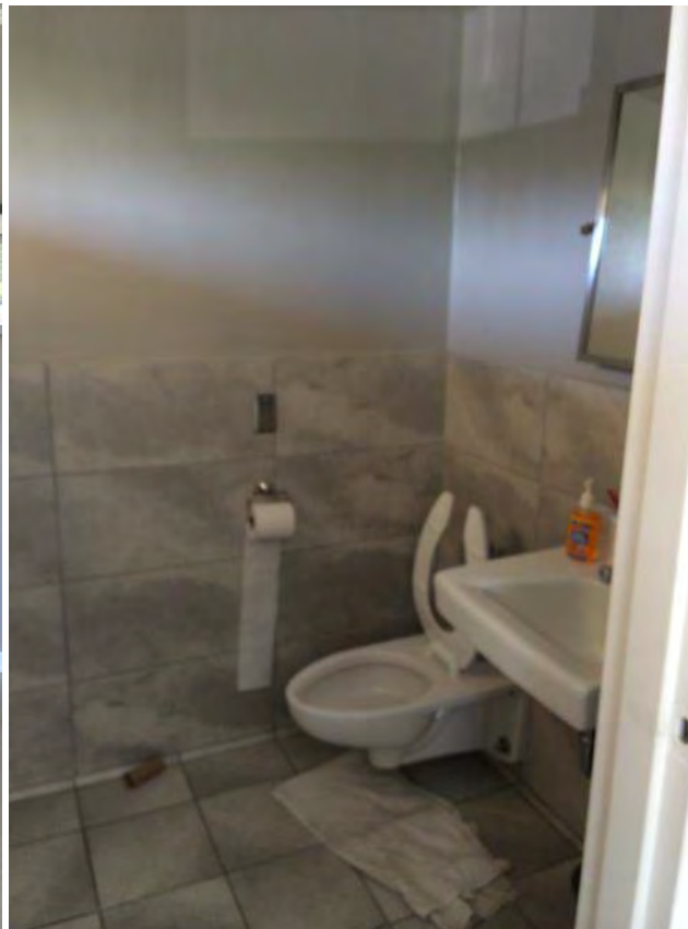
Tile toilet rooms, community showers
