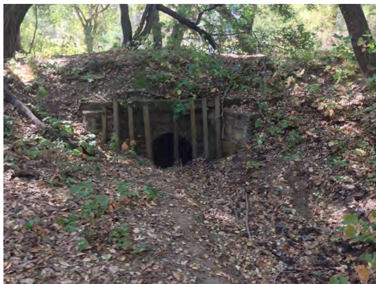
Photo 5: Culvert within tributary to Cordilleras Creek
