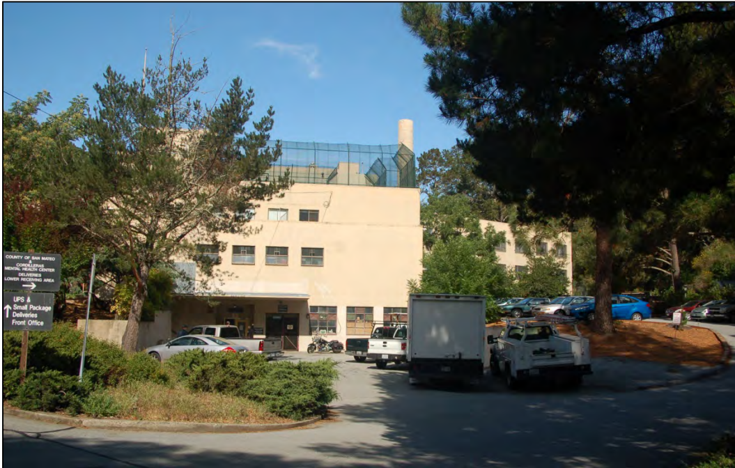
Main block, east façade – view to the west
