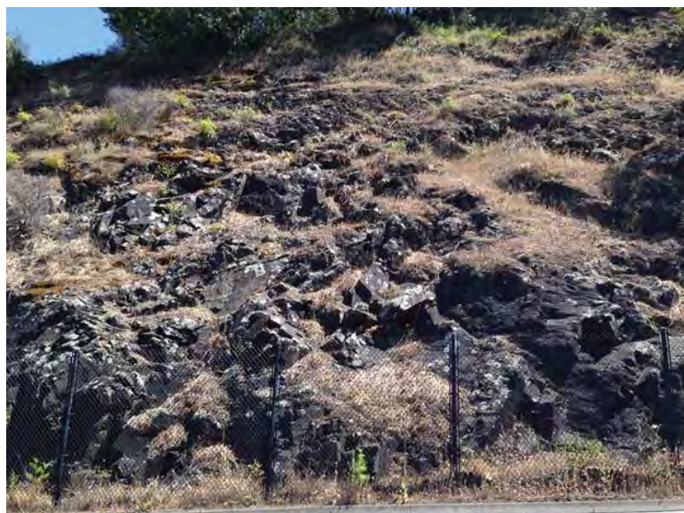
Photo 13: Road cut on Edgewood Road (southeast of site) composed of blocky sandstone
