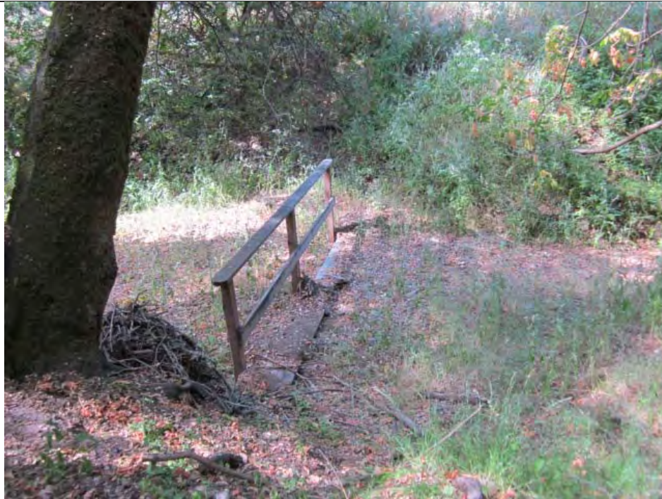
Photo 4: Structure in the creek bed.
