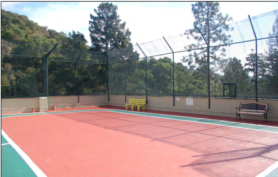
Third floor roof deck – view to the northeast
