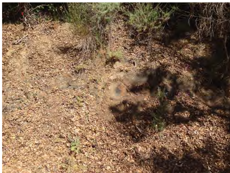
Photo 3: Cut slope behind water tank
