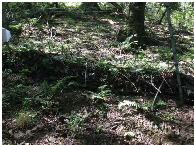
Photo 9: Rock and organic debris accumulation against site boundary fence
