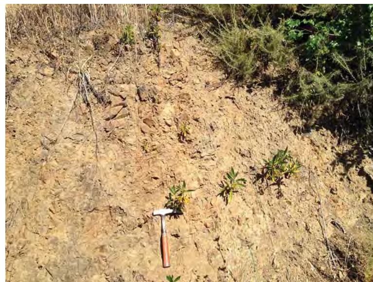
Photo 2: Cut slope beneath water tank
