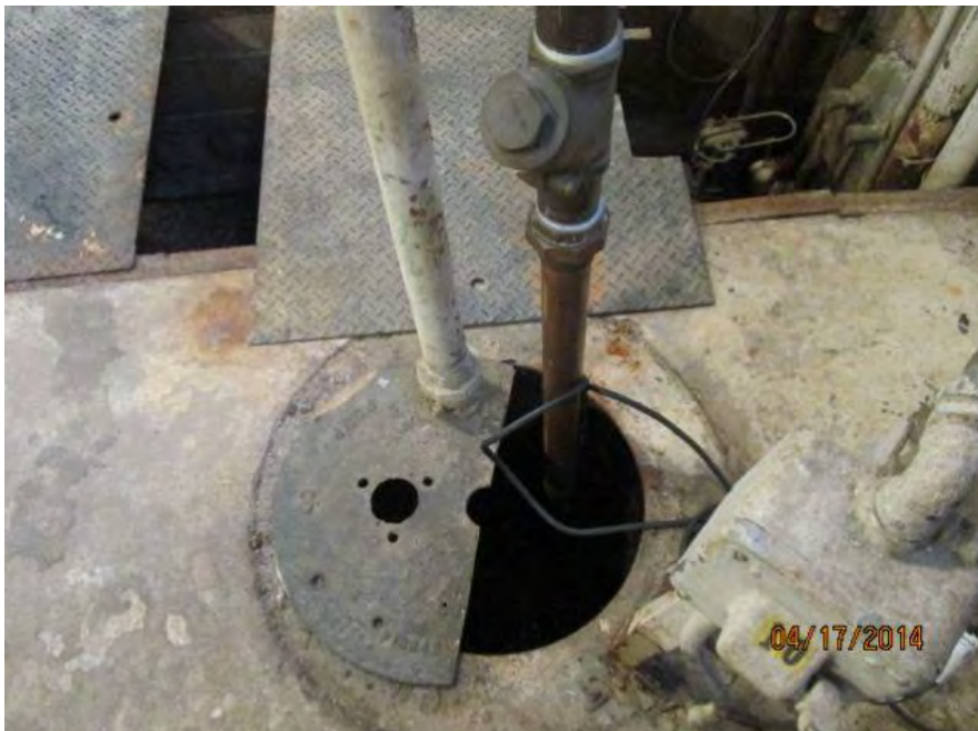
Photo P-4 - Sump Pit in Boiler Room
