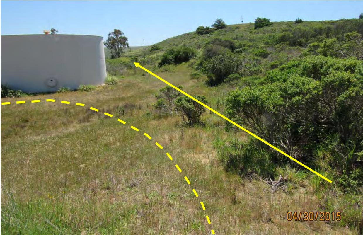
**Photo 4** – Photo of ephemeral drainage channel (solid arrow) adjacent to the proposed new storage tank location (dashed line). Note – drainage channel flows directly to the Quarry Pond, which is located adjacent to the trees shown in the photo background more than 200-feet from the construction area.
