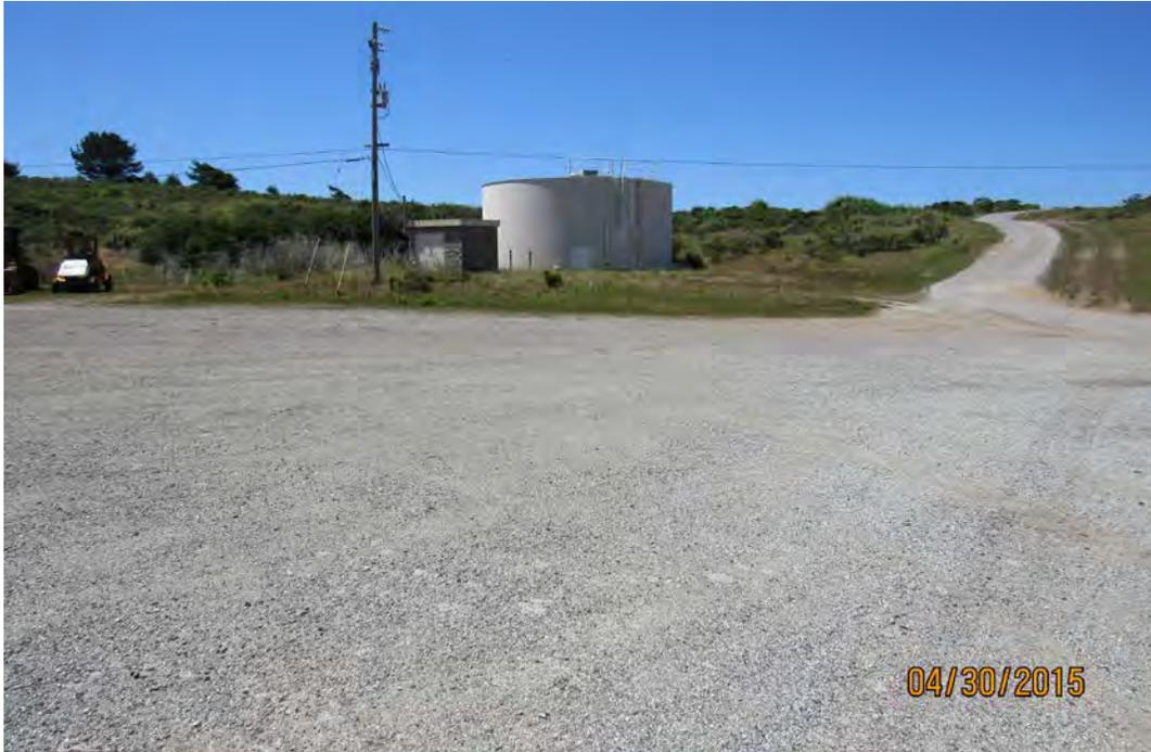
**Photo 2** – Photo of project site, including: staging and temporary material storage area (foreground), existing chlorine building and water storage tank (background), proposed location of new water storage tank (right of existing tank), and proposed location of new well (in front of existing tank).
