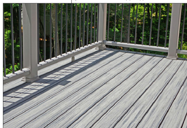
ALL DECKING: COMPOSITE BRAND: TREX COLOR: ISLAND MIST RAILING: COMPOSITE/ALUM. BRAND: TREX COLOR: GRAVEL PATH POSTS W/ BLACK ALUM. BALUSTERS
