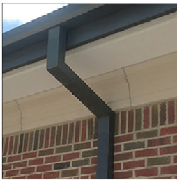
GUTTER & DOWNSPOUTS: ALUM. BRAND: DREXEL METALS, OR EQ. COLOR: MEDIUM BRONZE
