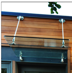
ENTRY AWNING: GLASS HARDWARE: CR LAURENCE COLOR: STAINLESS STEEL
