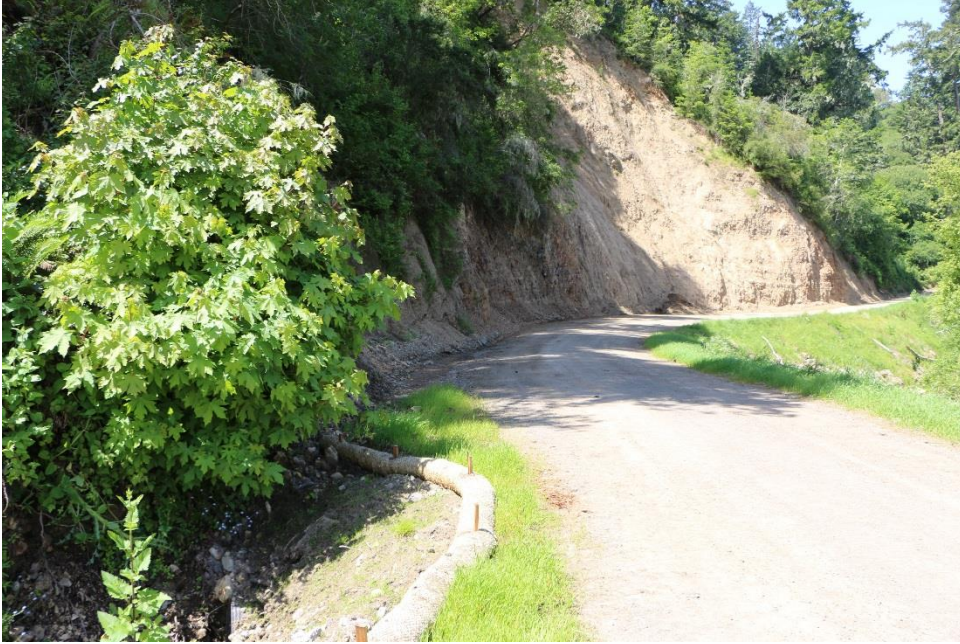
Landslide area adjacent to San Gregorio Creek
