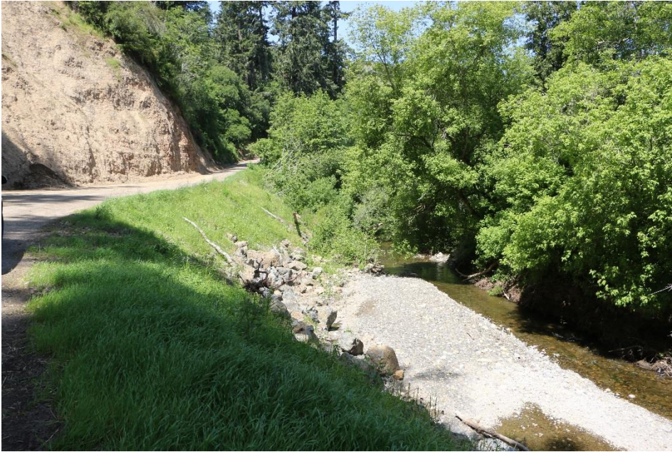
San Gregorio Creek bank stabilization
