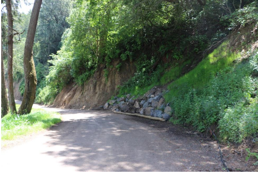
Example of slope stabilization
