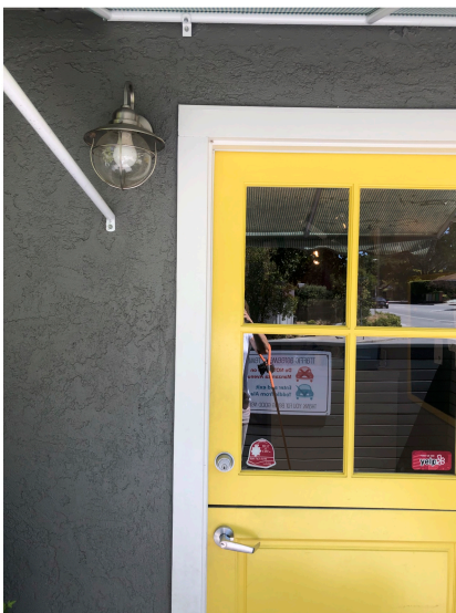
North side of the structure facing Manzanita Avenue
