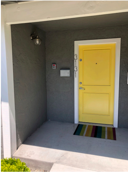
West side of structure facing Alameda de las Pulgas
