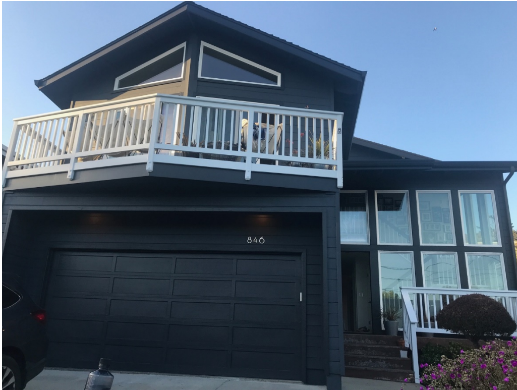
Front of existing residence. New front wall to be painted to match the existing main body and trim colors. The roof modification at the front to be patched with composition shingle roofing to match the existing roofing.
