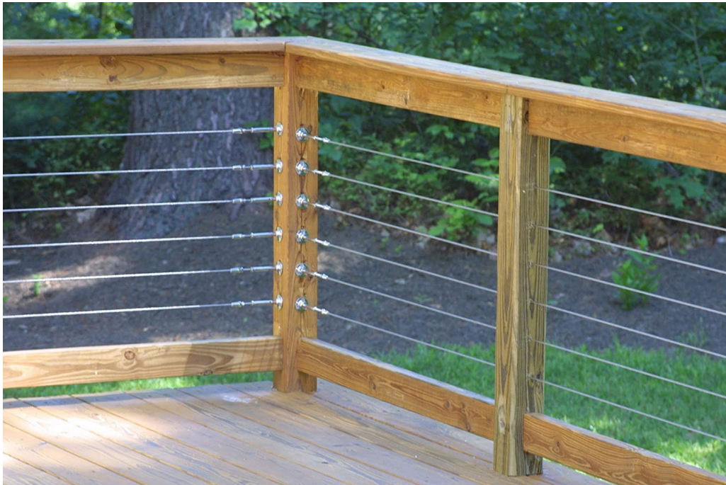
Proposed cable railing system at existing front deck. Wood components of railing to be painted to match the existing deck post color.
